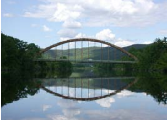
The historic Samuel Morey Bridge links Orford and Fairlee.
