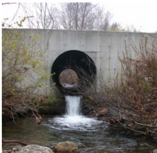
A hanging culvert at the Dartmouth Skiway obstructs fish passage.
