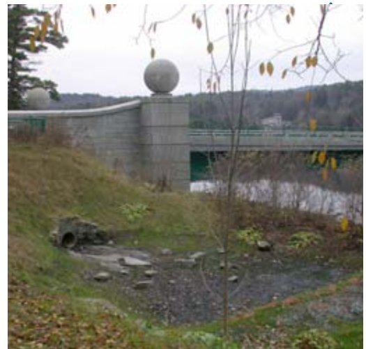
Stormwater from West Wheelock St. in Hanover is detained and cleaned here, not delivered directly to the river.
