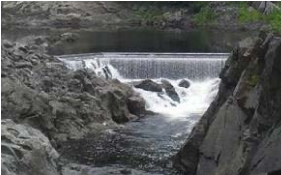
Photo: Low-head Dam in Bellows Falls Bypassed Reach.
