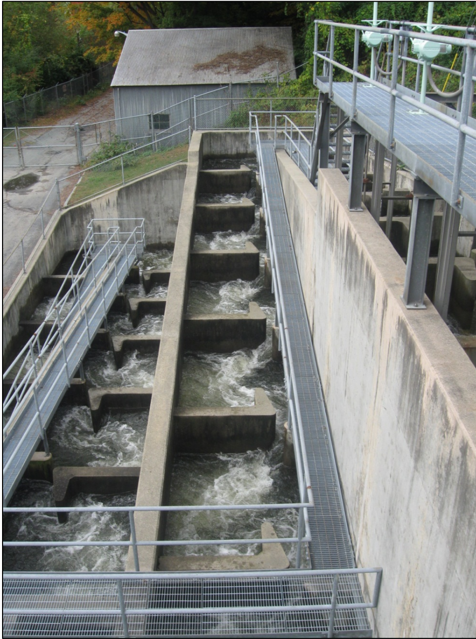
Figure A-9. Upstream fish passage facilities.
