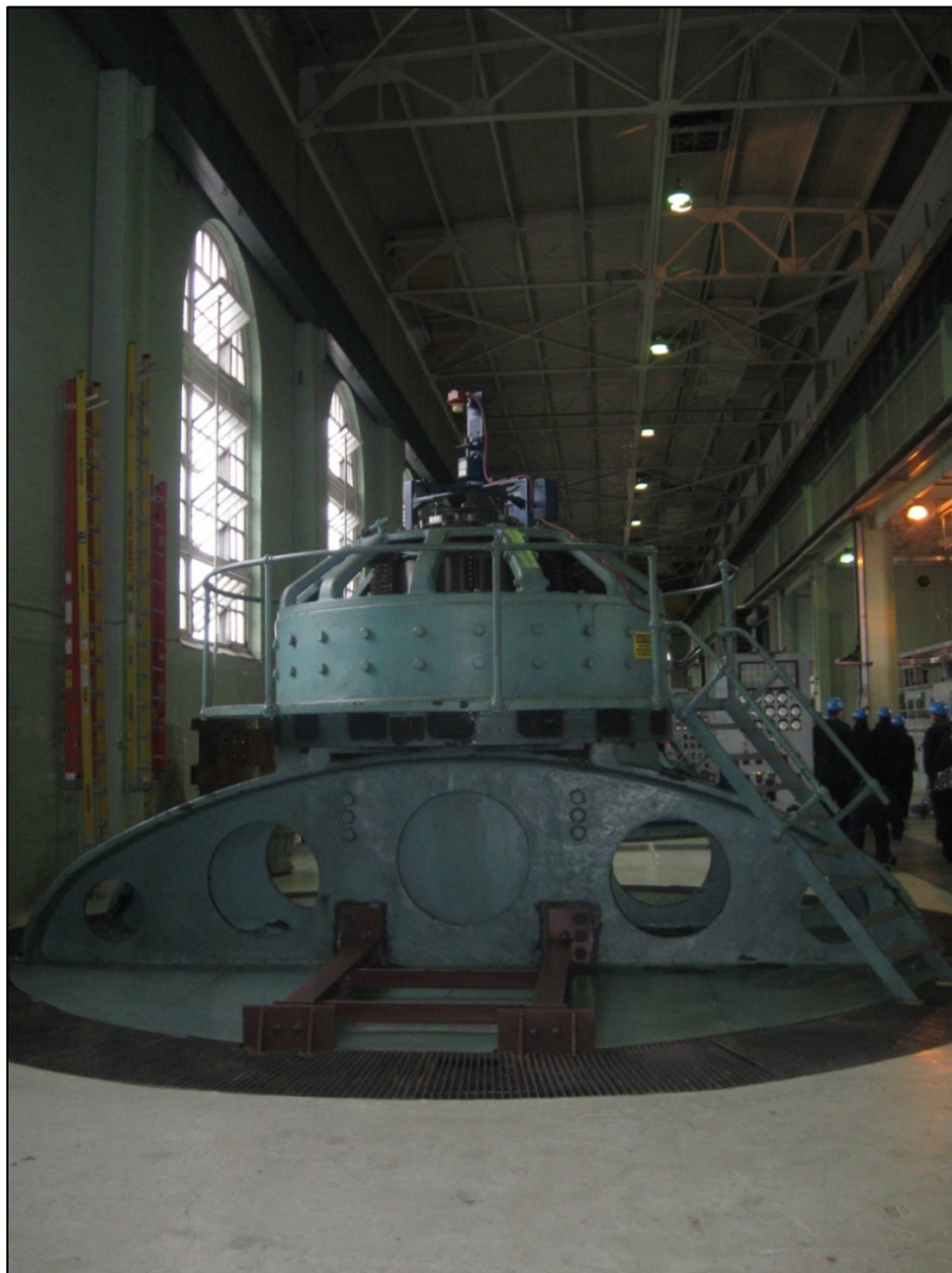
Figure A-4. Powerhouse, Unit No. 10.
