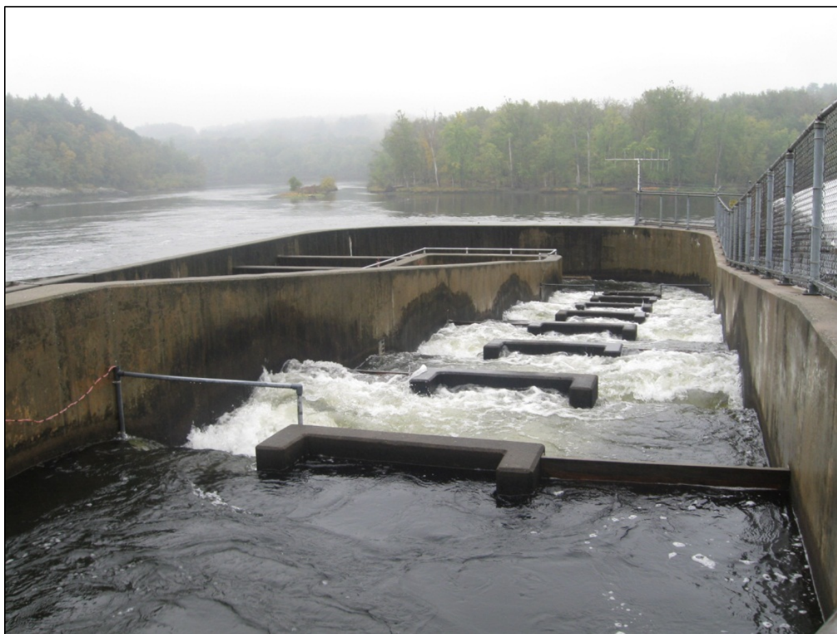
Figure A-6. Upstream fish passage facilities.
