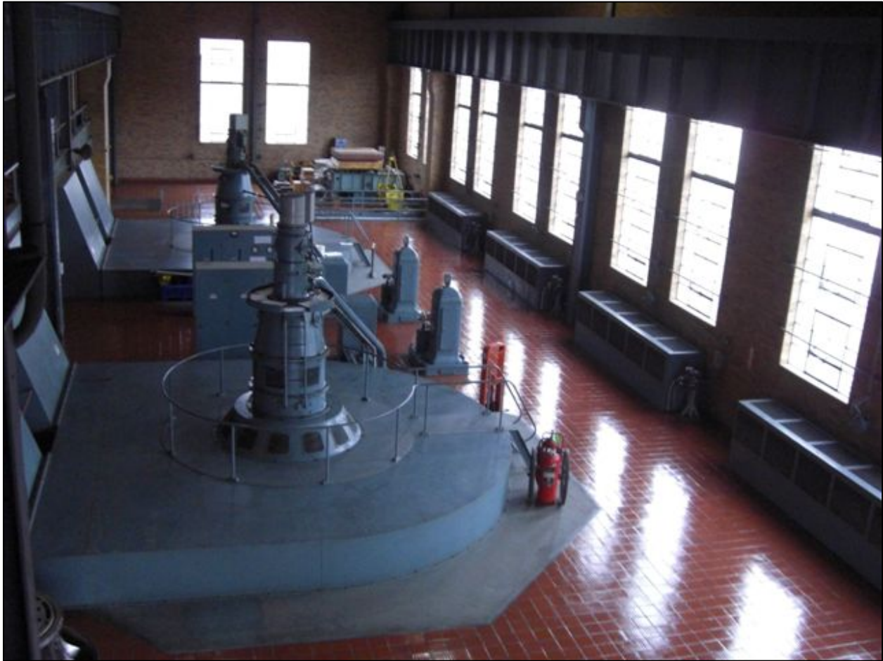
Figure A-4. Unit No. 1 (foreground) and Unit No. 2 (background).
