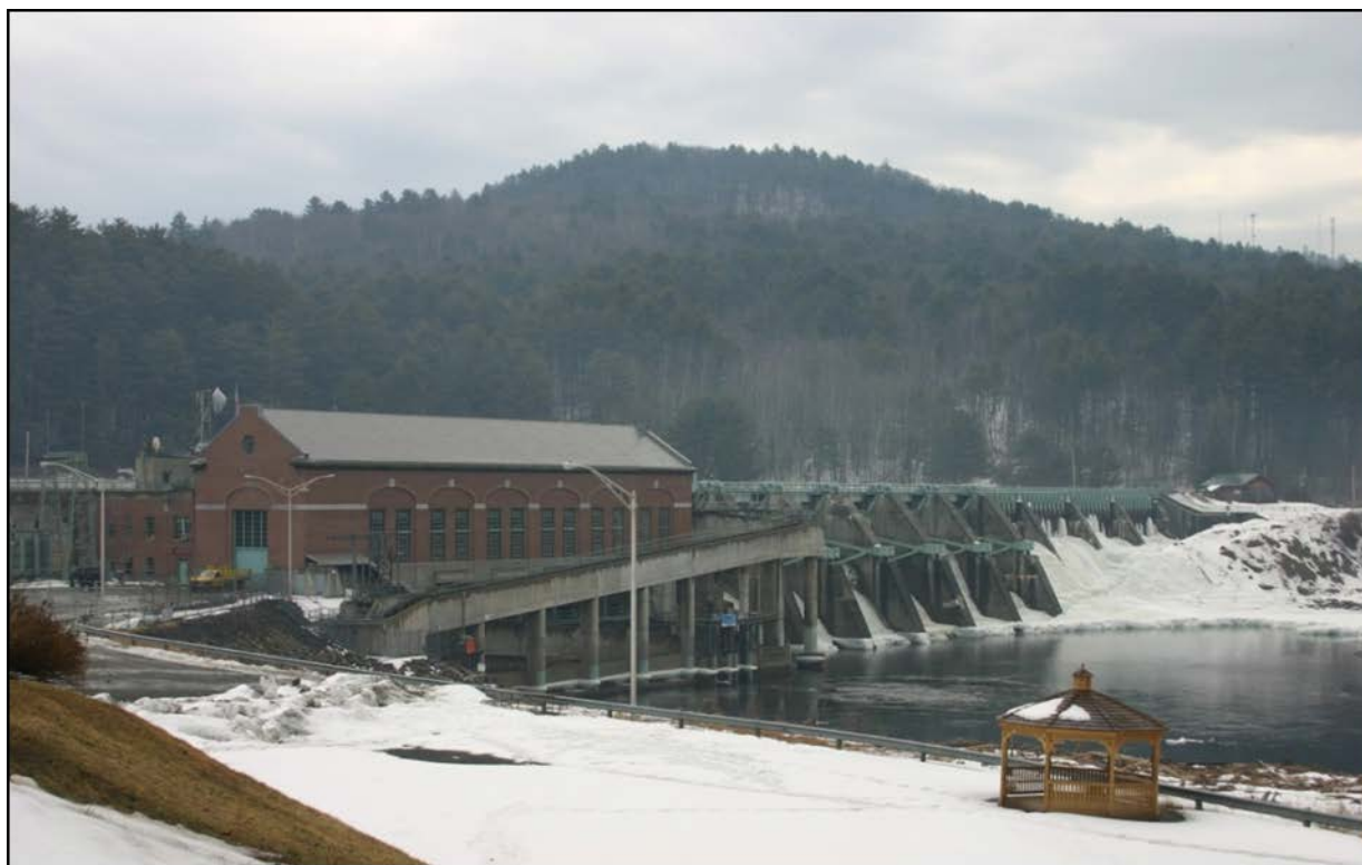
Figure A-2. Powerhouse, dam, and fish ladder.
