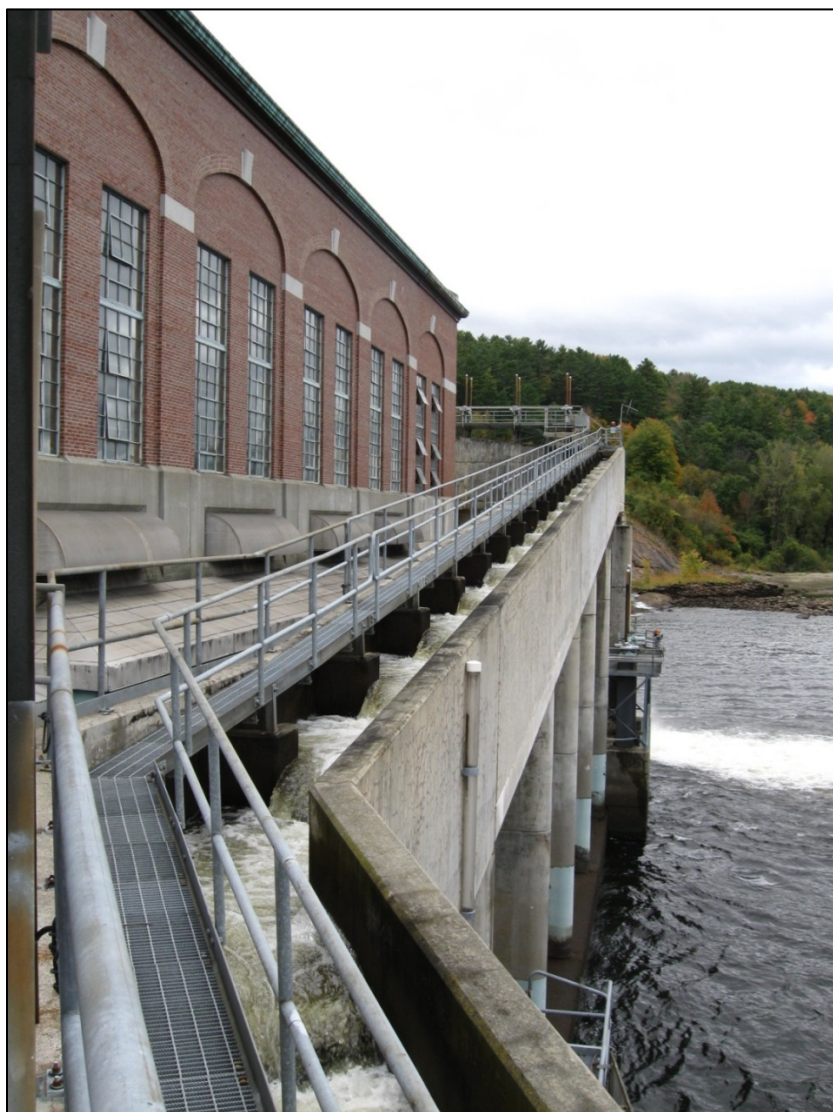
Figure A-6. Upstream fish passage facilities.
