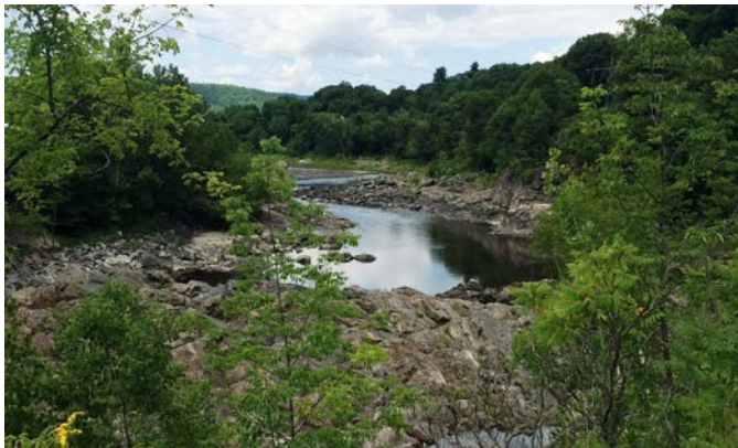
KOP 3 – Demo Flow 1 Upstream (US) (125 cfs)
