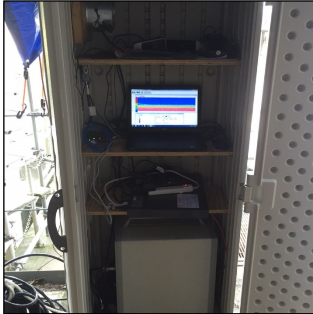
Figure 3.2.2-1. Equipment cabinet with laptop computer, communications hardware, uninterruptible power supply, and HTI Model 243 echosounder.
