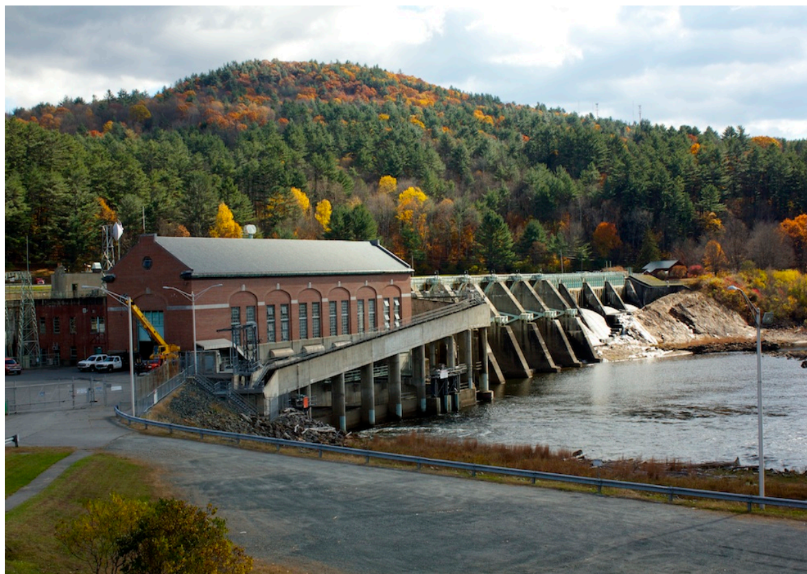
Wilder Dam in October 2012.
