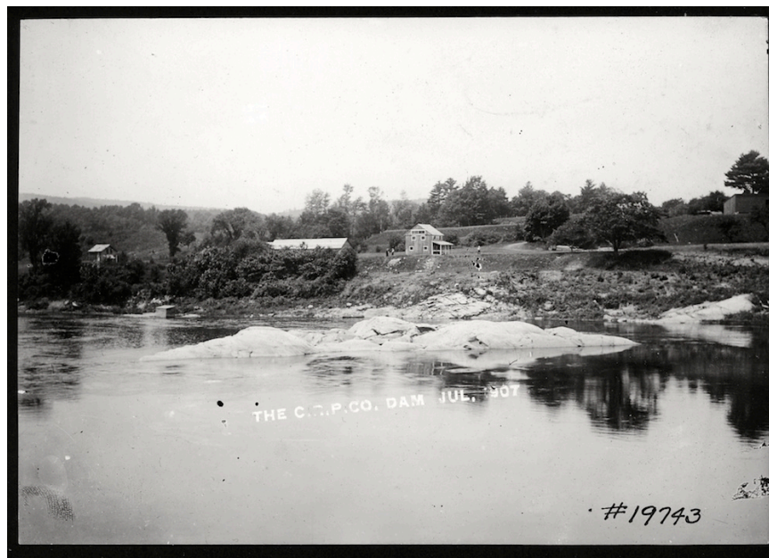
Vernon Rapid Before the Dam--1907
