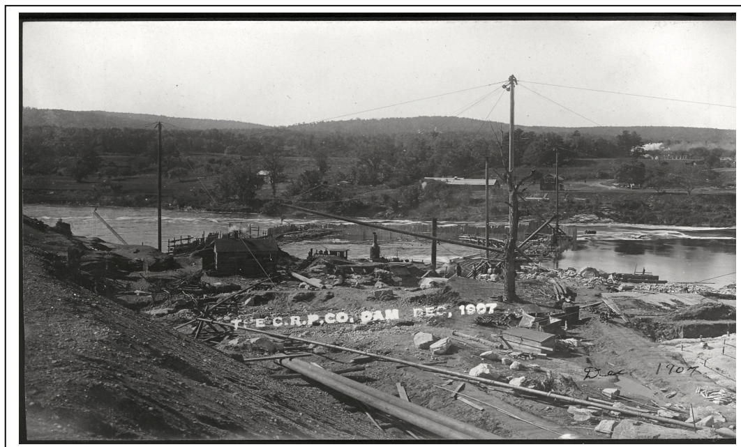
1907 Dam Construction—Note Whitewater Rapids in Background Soon To Be Lost
