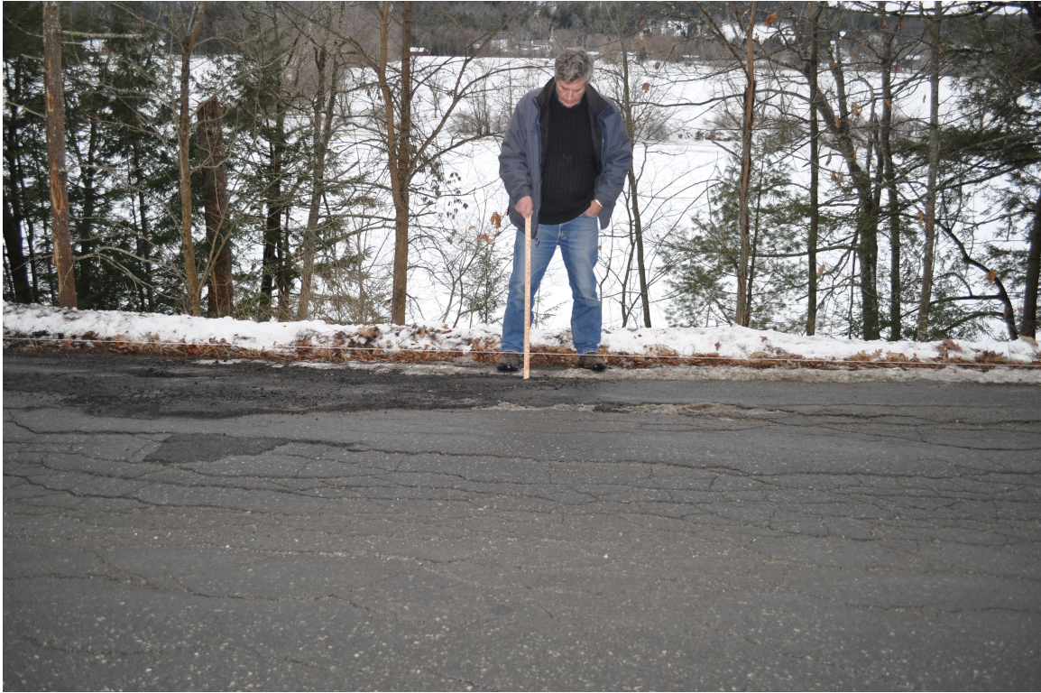
Figure 4. River road south looking west. Wilder impoundment in background. Slump in road is 7 inches.
