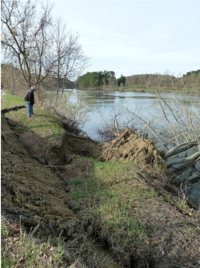
Figure 1. Collapse of a portion of Wilder impoundment bank in spring of 2011 necessitating reconstruction of 1200 feet of River Road south of its intersection with the North Thetford Road in Lyme , New Hampshire.
