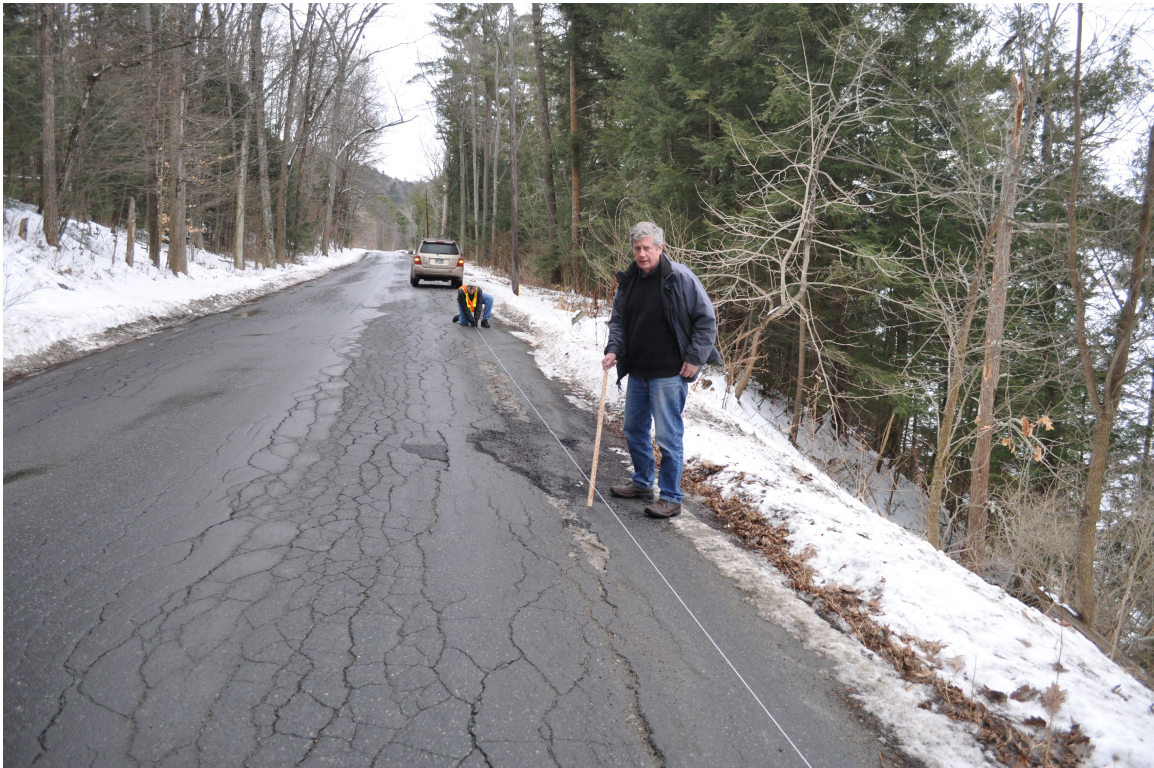
Figure 3. River Road, Lyme, looking south about a quarter mile south of the East Thetford bridge. The string is on the road at each end of the slump which is 7 inches below the string in the center. Note the cracking of the blacktop on the west side of the road due to the slump and compare it with the cracking seen in the photo taken at the site of the collapse near the North Thetford road in figure 2
