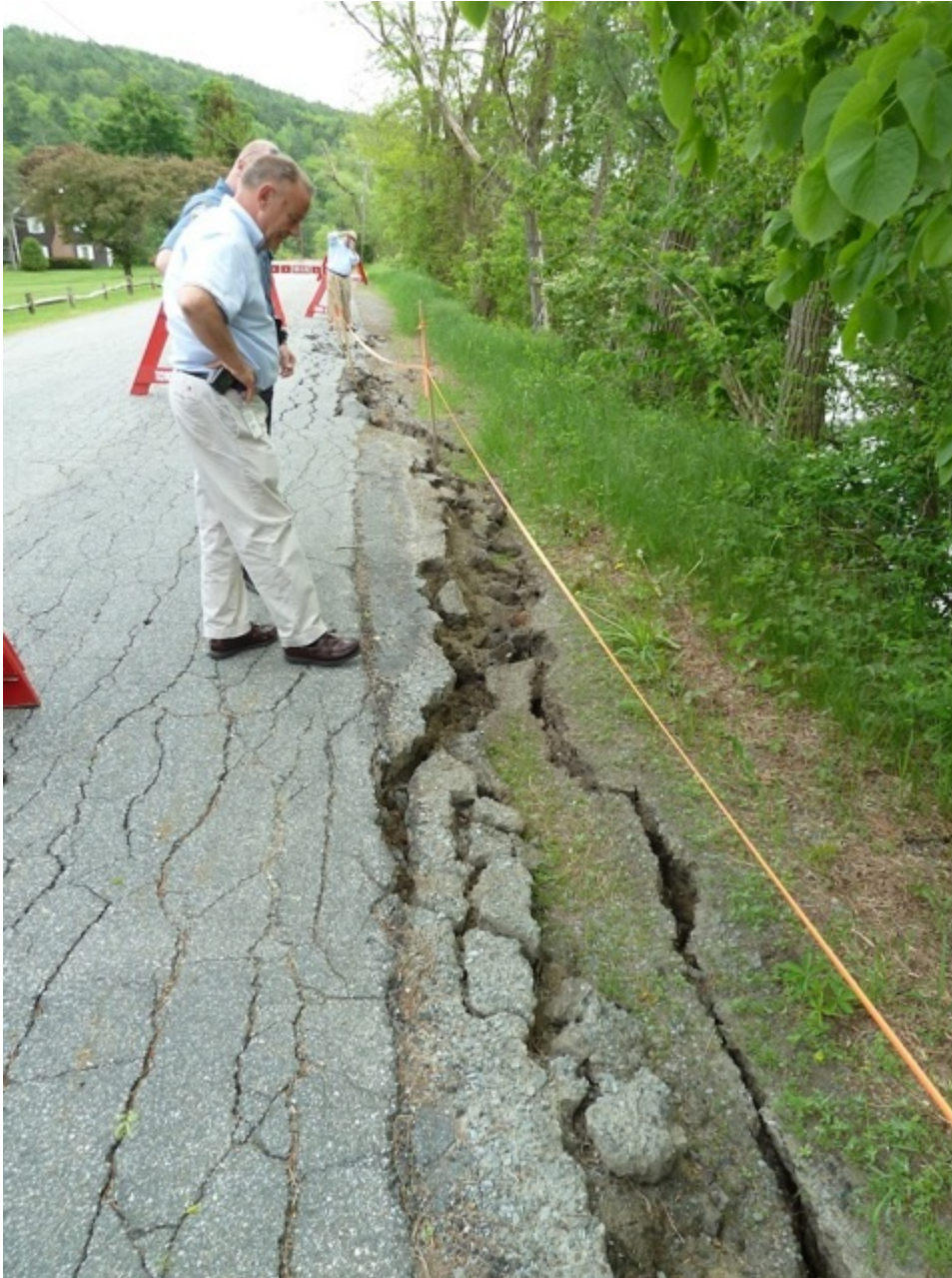
Figure 2 River Road north adjacent to bank collapse. Note pattern of cracks in blacktop and compare with those in photo 3, below, in area of slumping River Road South.
