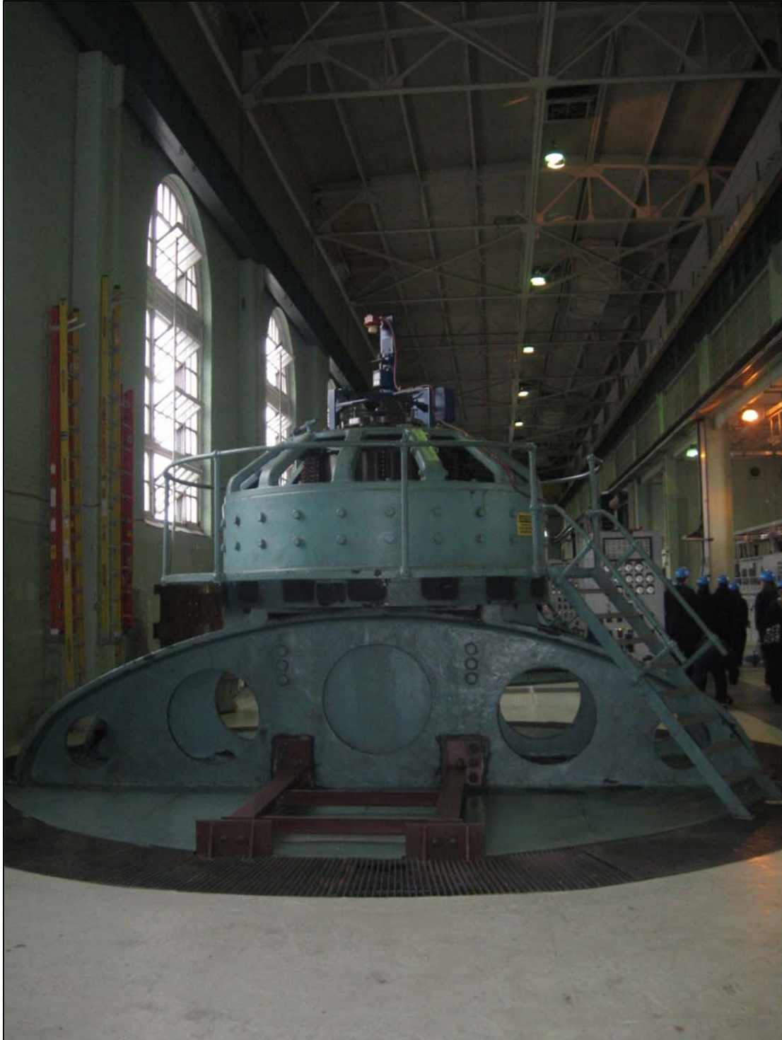
Figure 2.3-3. Generator Unit No. 10.
