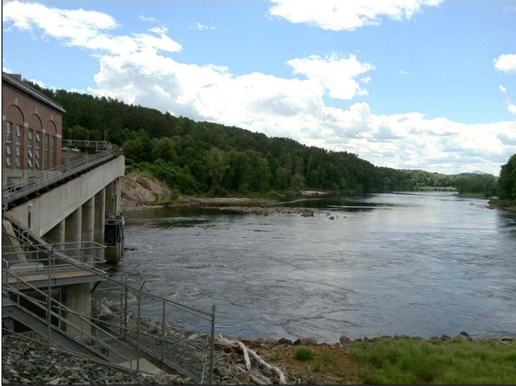
Figure 3.11-1. View downstream of Wilder dam.
