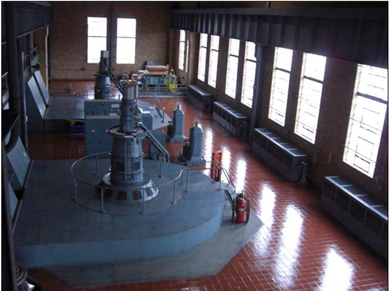
Figure 2.3-3. Generator Units No. 1 and 2.
