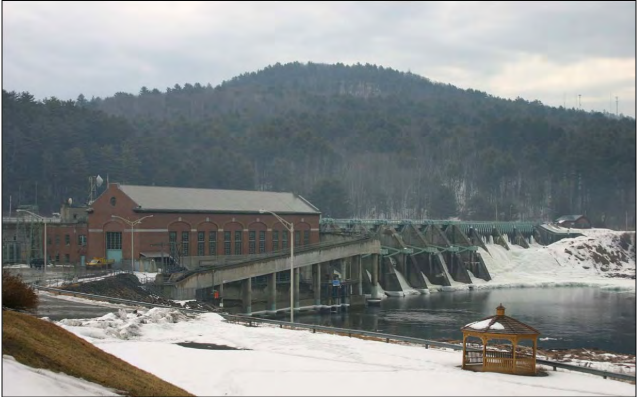
Figure 2.3-1. Powerhouse, dam, and fish ladder.
