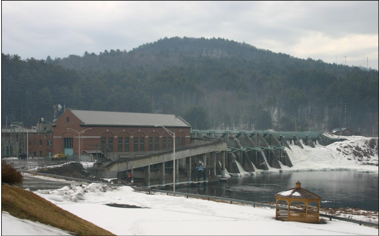
Figure 2.3-1. Powerhouse, dam, and fish ladder.
