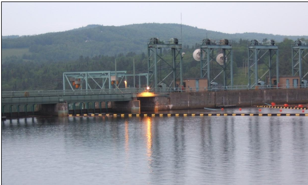
Figure 2-4. Moore fish trap forebay attraction light. The skimmer gate attraction light is not visible from this angle.
