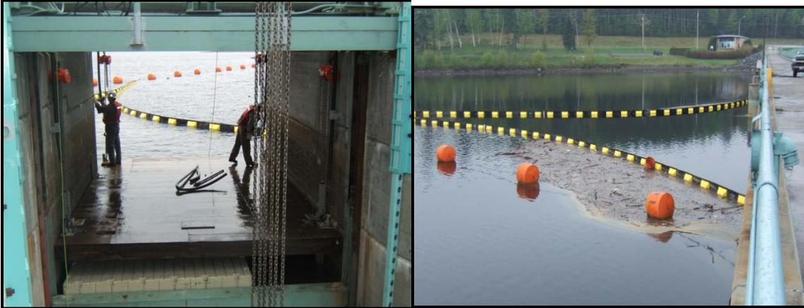
Figure 2-3. Moore Development, attraction flow shelf raised for repairs (left); view is looking upstream through the skimmer gate entrance to Moore Reservoir and the debris boom (right).
