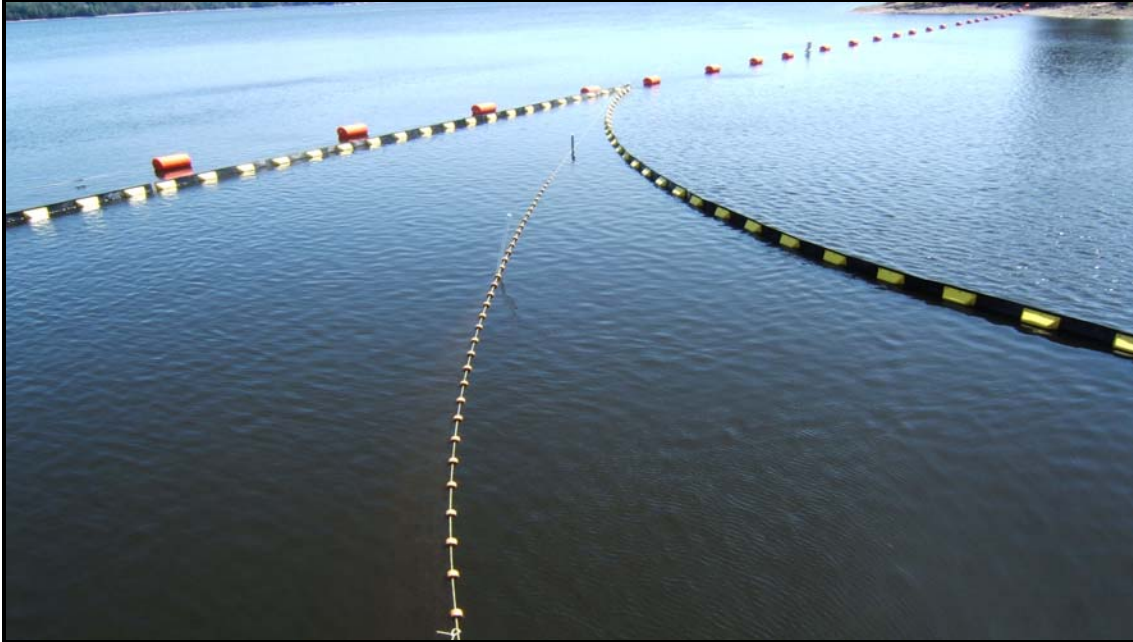
Figure 3-4. Guide net installed perpendicular to the fish sampler entrance (i.e., skimmer gate entrance) at Moore Dam, spring 2009.
