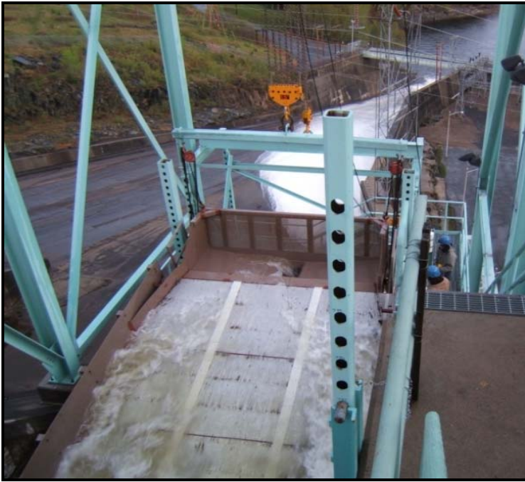
Figure 2-2. Dewatering surface of the Moore Development fish sampler.
