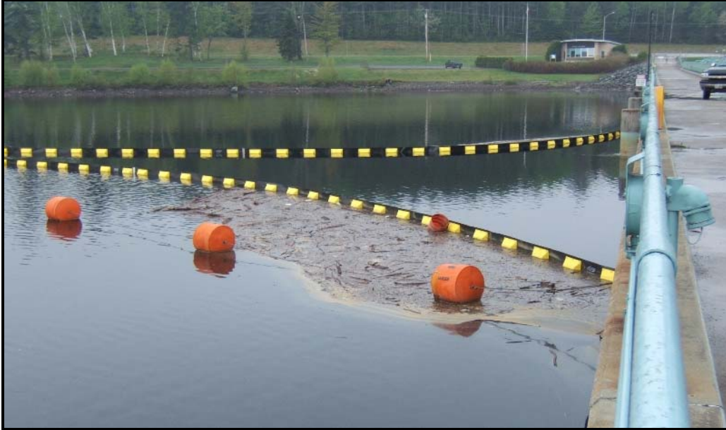
Figure 2-6. Moore Dam trash boom installed at the entrance to the skimmer gate.
