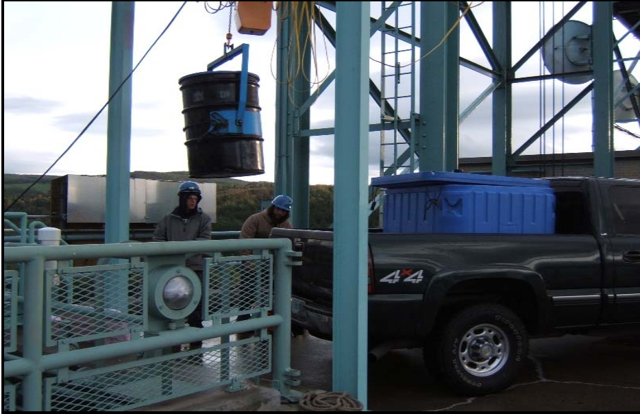
Figure 3-2. Moore Development, monorail system used to transport fish from the sampler collection tank to the transport tank.
