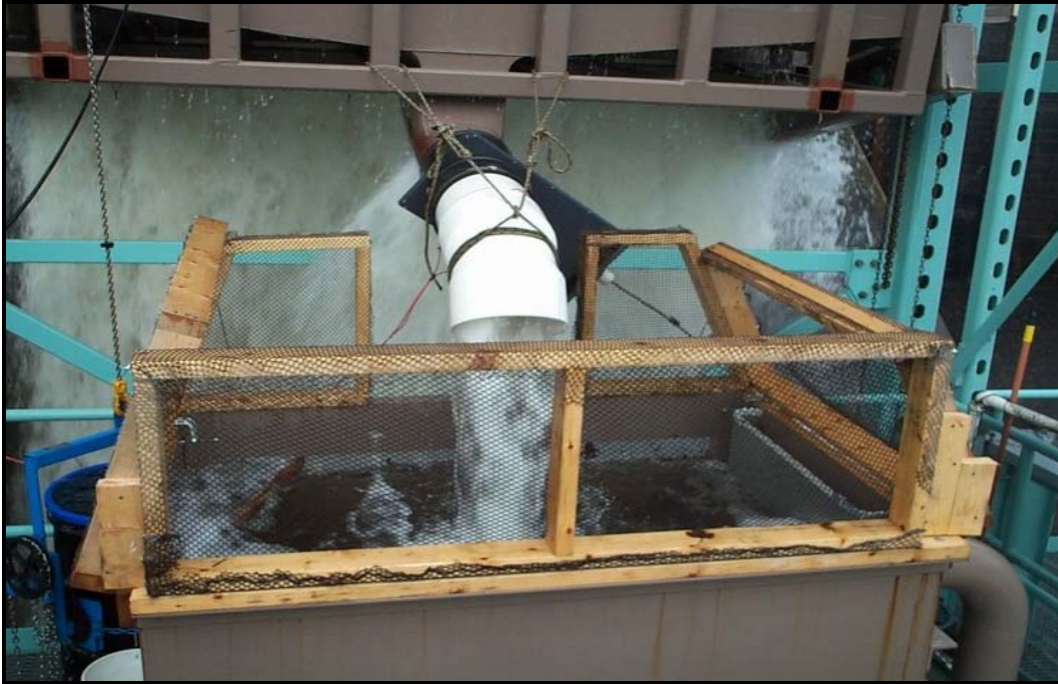
Figure 2-4. Downstream end of the Moore fish sampler in fishing mode, showing the discharge pipe and collection tank.
