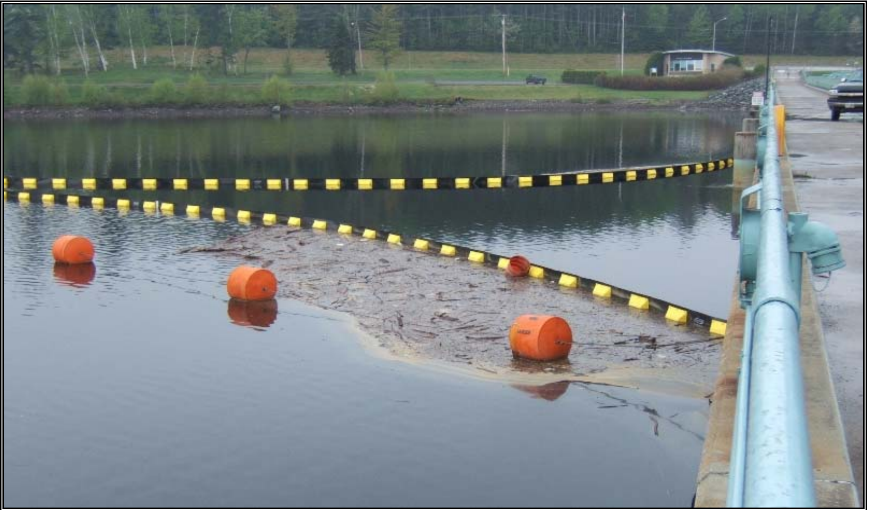
Figure 2-1. Moore Dam trash boom installed at the entrance to the skimmer gate.
