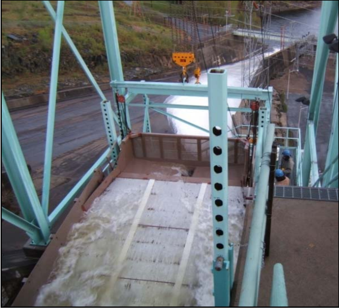
Figure 2-4. Dewatering surface of the fish sampler at Moore Dam.
