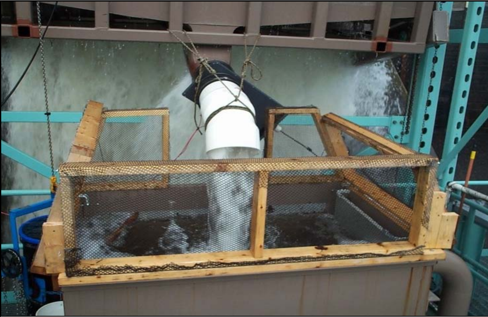
Figure 2-6. Downstream end of the Moore Dam fish sampler in fishing mode, showing the elbowed discharge pipe and collection tank.
