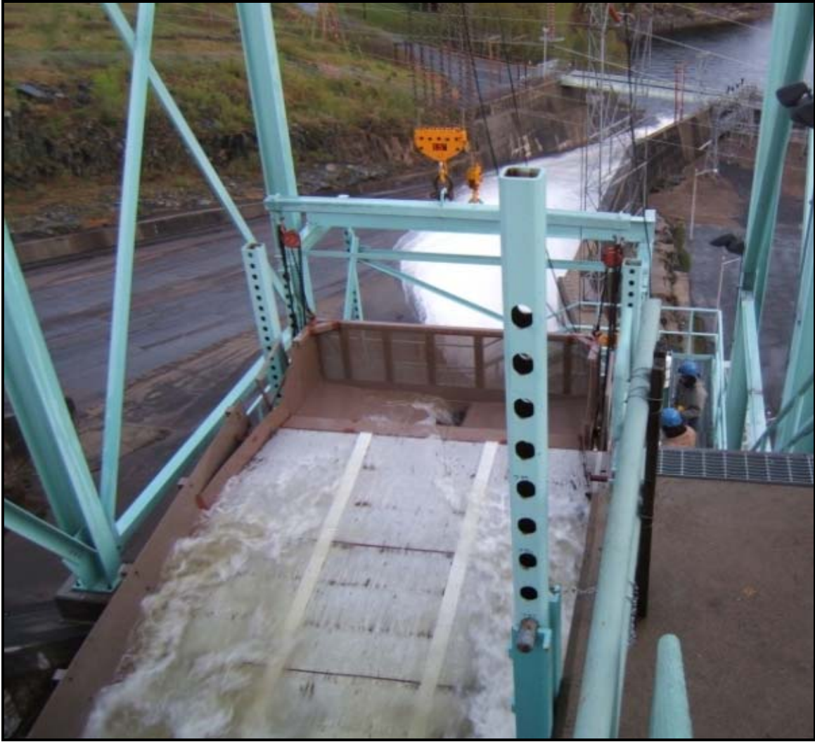
Figure 2-5. Dewatering surface of the fish sampler at Moore Dam.
