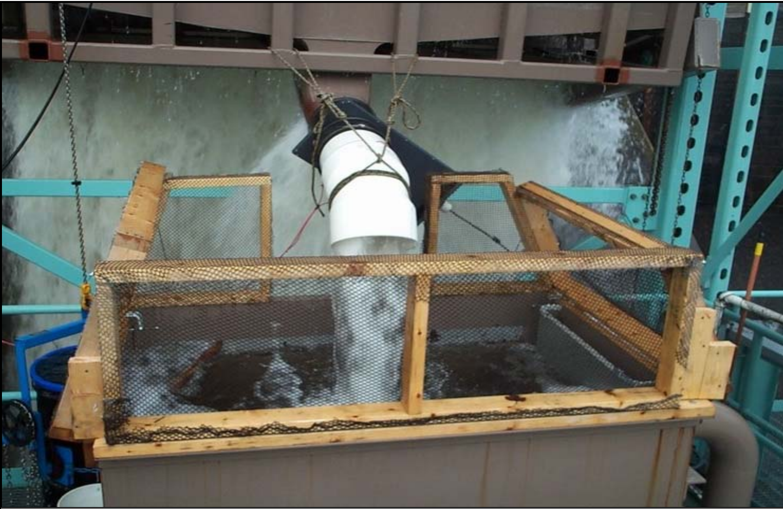
Figure 2-7. Distal end of the Moore Dam fish sampler in fishing mode, showing the elbowed discharge pipe and collection tank.
