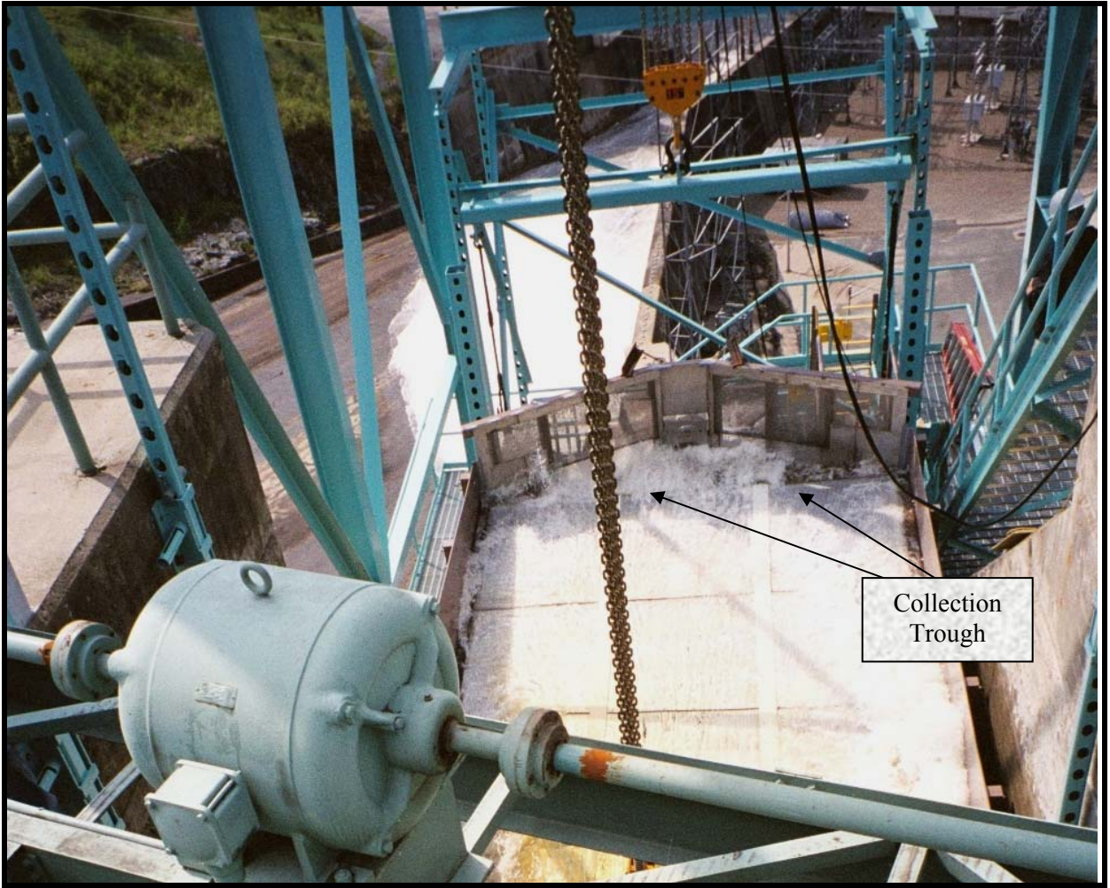
Figure 2-4. Moore Development, inclined plane sampler showing the collection trough.
