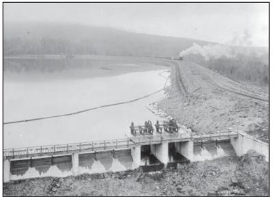
Somerset Development, Somerset, VT, built 1911–1913. View of 2,100-ft-long, 110-ft-high modified hydraulic earth fill dam looking south with spillway in foreground. Construction railway track and steam locomotive pulling dump cars are visible on dam crest (ca. 1913).
