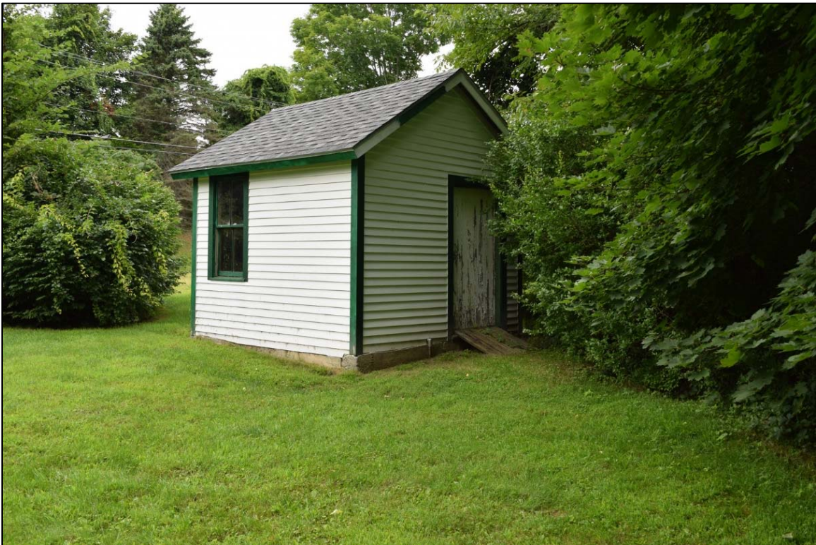
Photo 6-11. Vernon Project, Hoister House, looking northwest.
