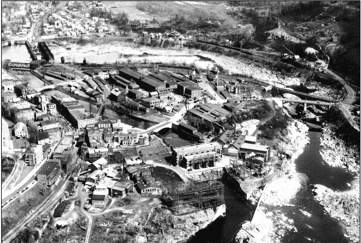
Figure 5-5. Circa 1932 aerial view of the Bellows Falls Project, looking north. Dam is at upper left and Canal extending from Dam to Powerhouse is at lower center.
