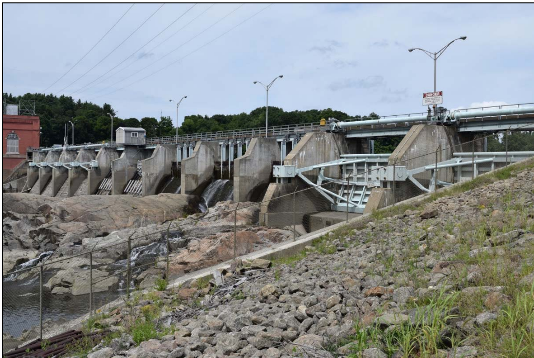
Photo 6-4. Vernon Project, Dam spillway looking northwest.
