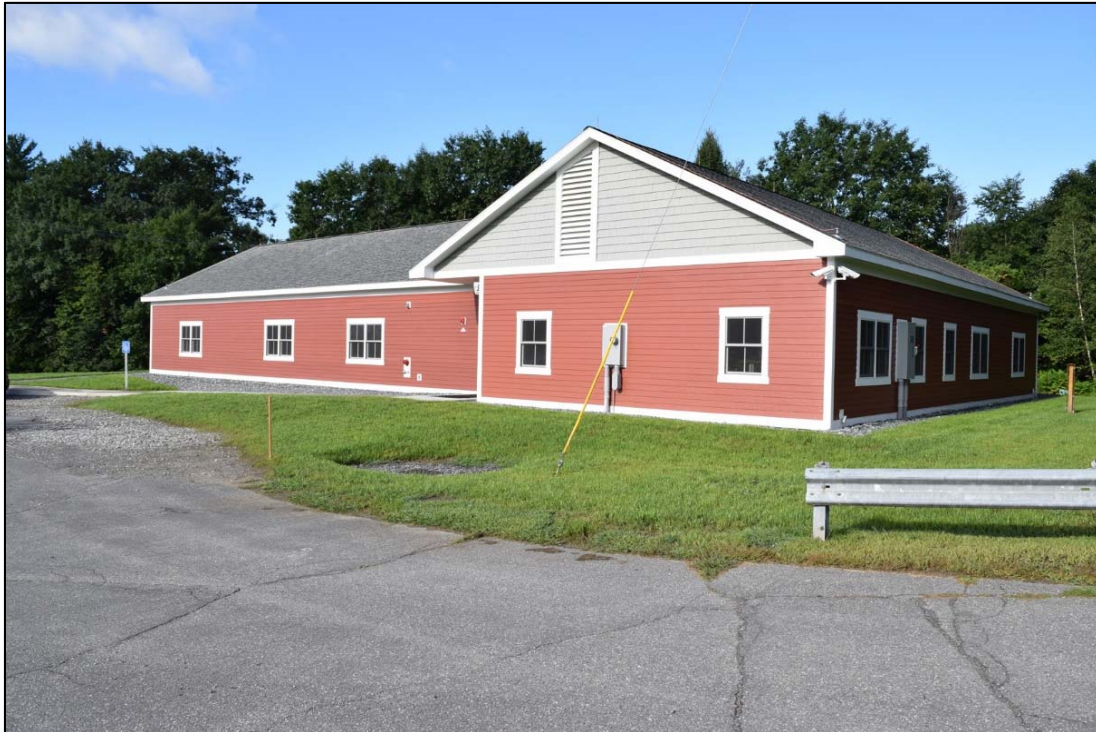
Photo 4-16. Wilder Project, Consolidated Control Center (CCC), looking southwest.
