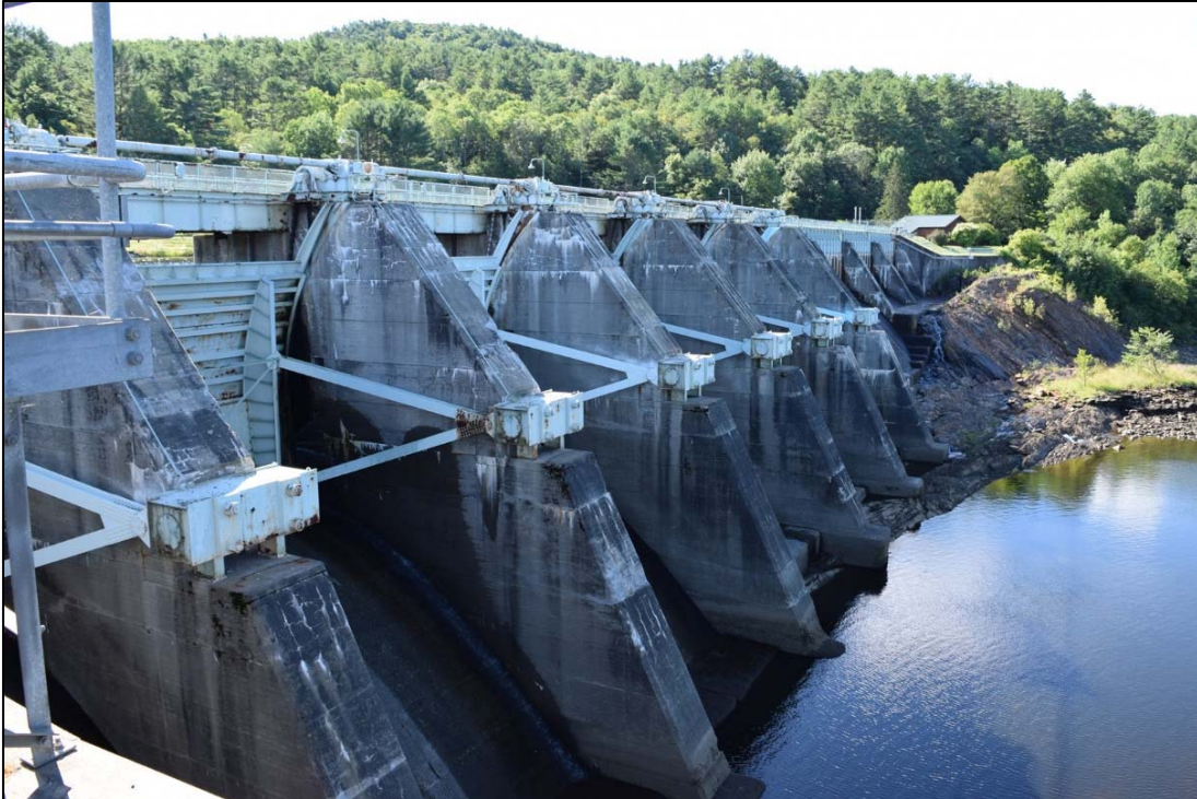
Photo 4-6. Wilder Project, Dam spillway, looking south.
