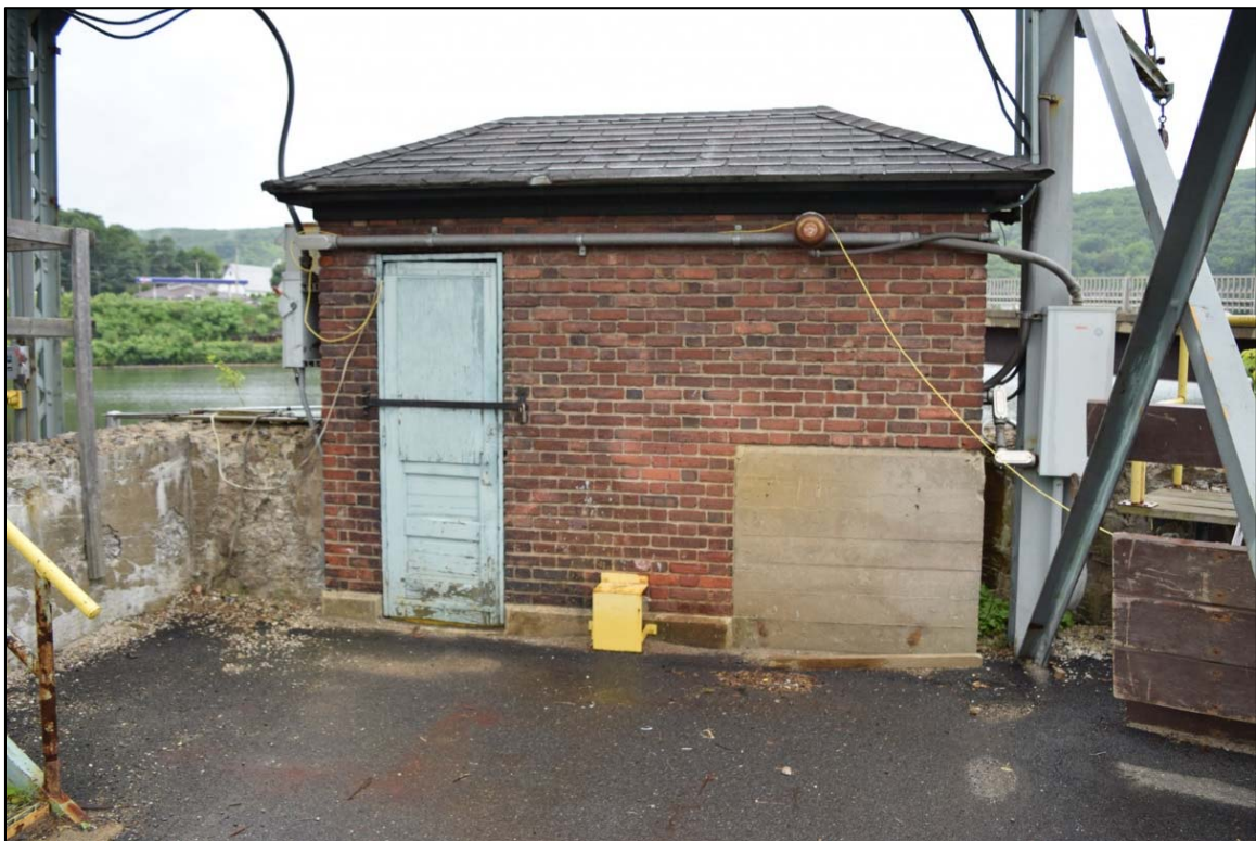
Photo 5-18. Bellows Falls Project, Gauge House, looking west.
