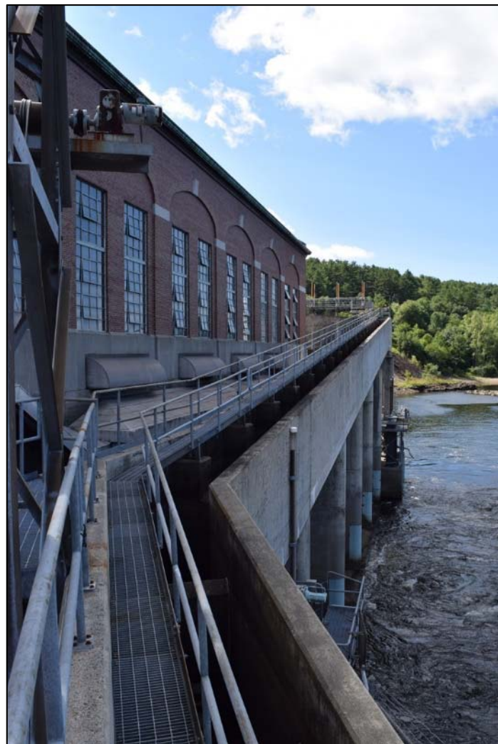
Photo 4-10. Wilder Project, Fish Ladder, looking south.
