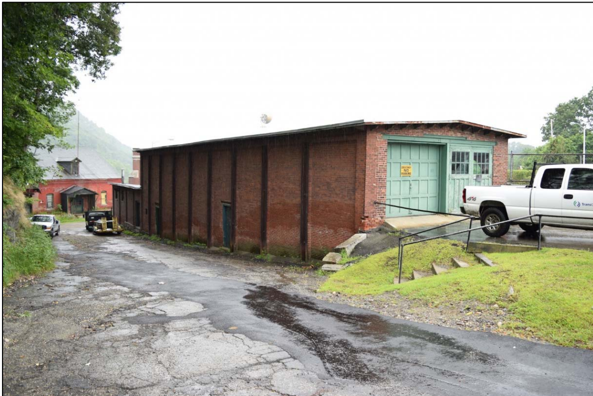
Photo 5-17. Bellows Falls Project, Six-Man Garage, looking southwest.
