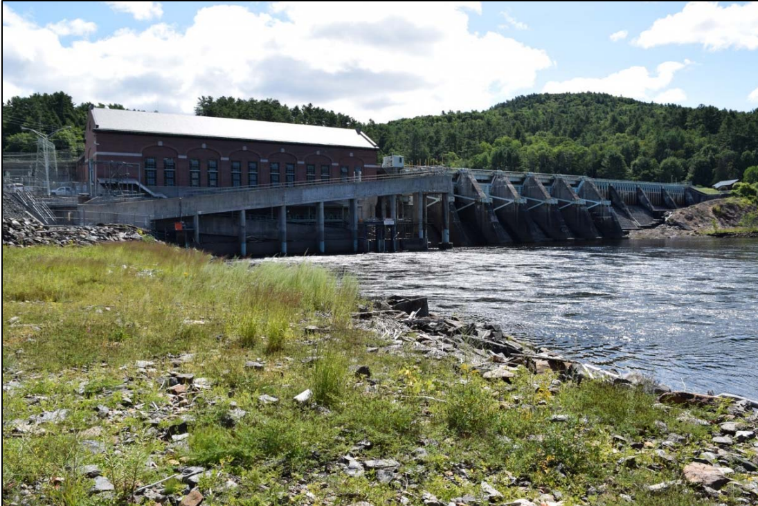
Photo 4-4. Wilder Project, Dam and Powerhouse, looking east from Vermont shore.
