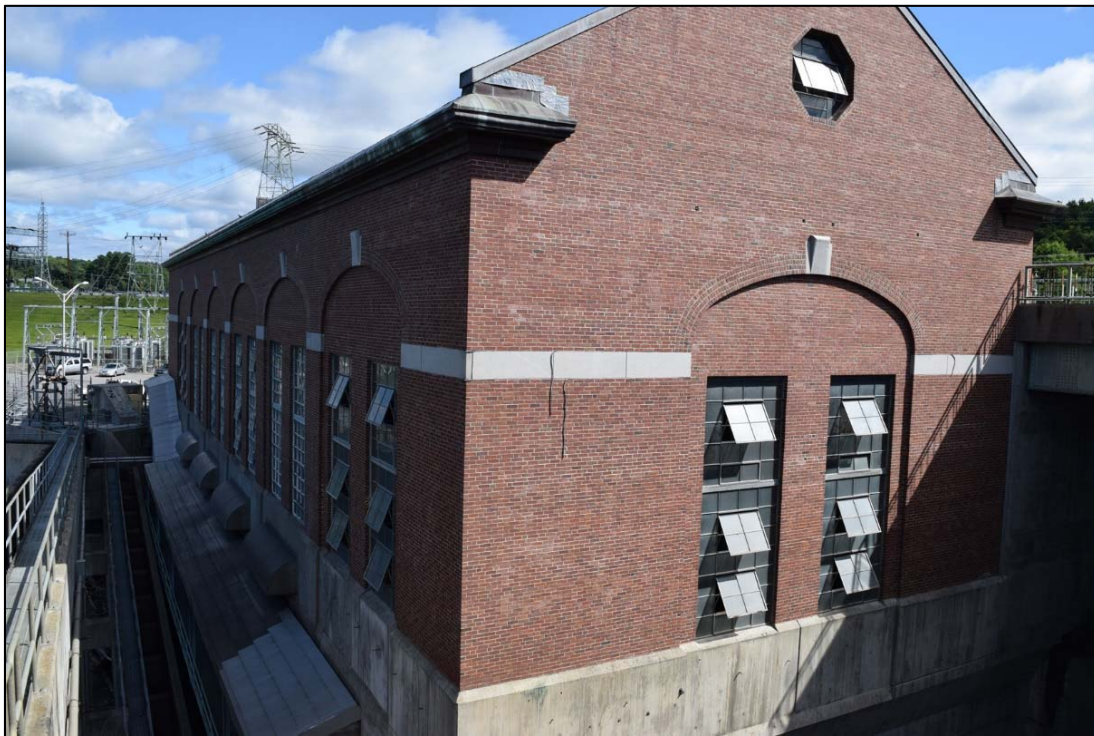
Photo 4-9. Wilder Project, interior of Powerhouse at generator floor, looking south.
