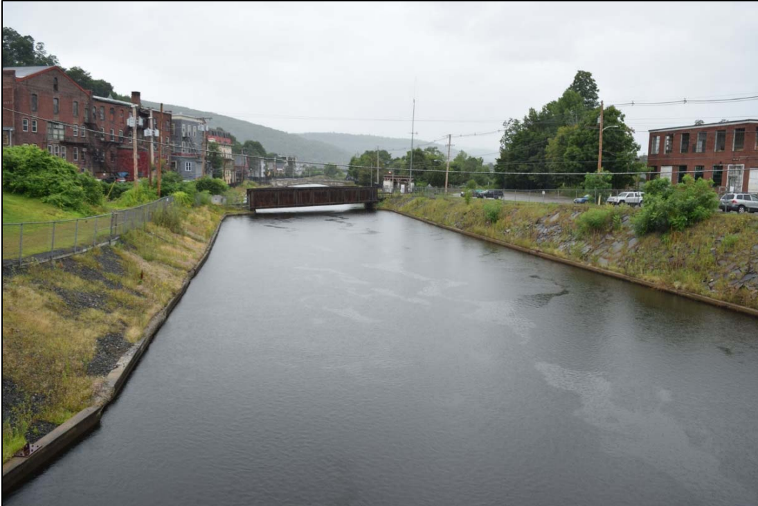
Photo 5-5. Bellows Falls Project, downstream end of Canal, looking north.
