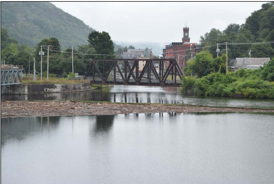
Photo 5-4. Bellows Falls Project, upstream end of Canal, looking south.
