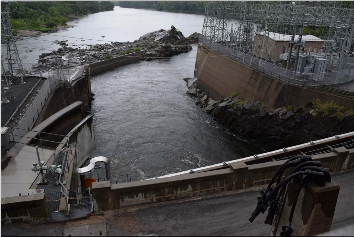
Photo 5-14. Bellows Falls Project, Tailrace, looking south from Powerhouse.
