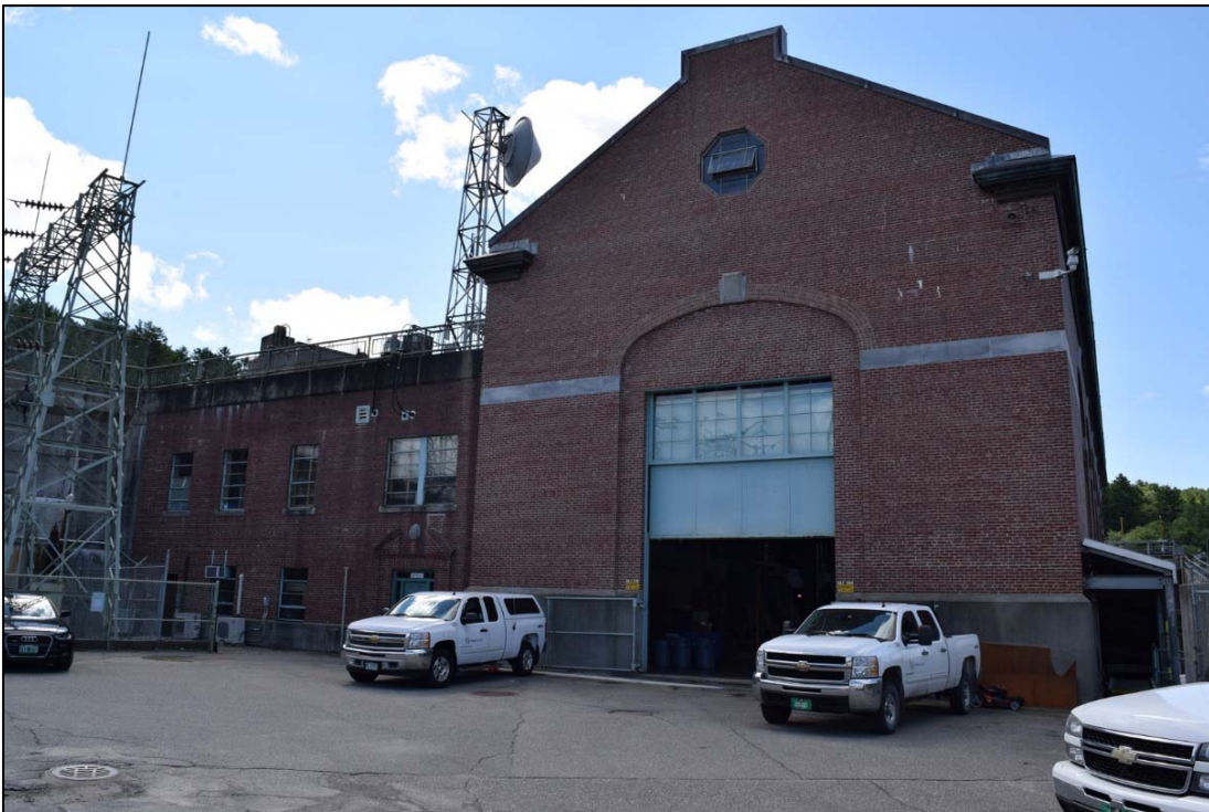
Photo 4-7. Wilder Project, north end of Powerhouse, looking south.
