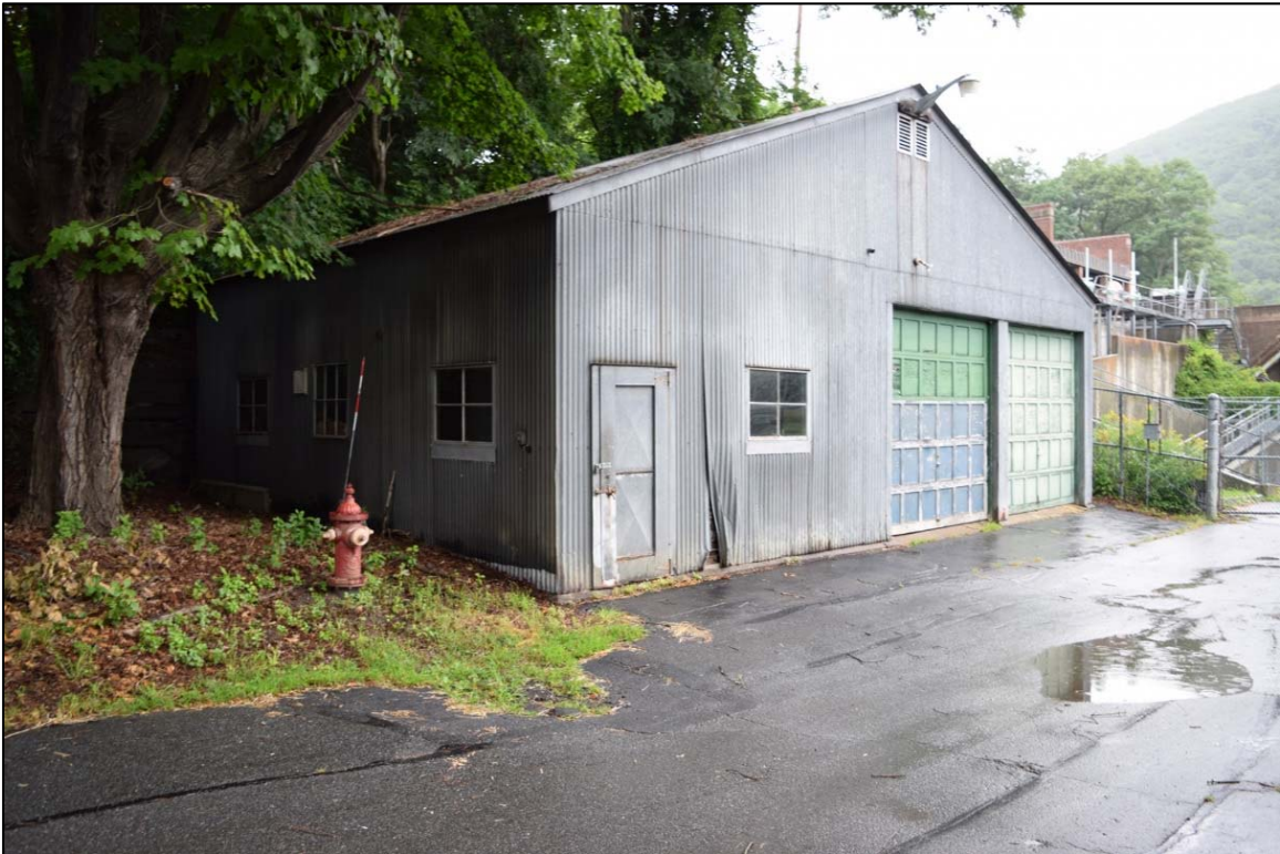
Photo 5-16. Bellows Falls Project, Line Shed looking northeast.
