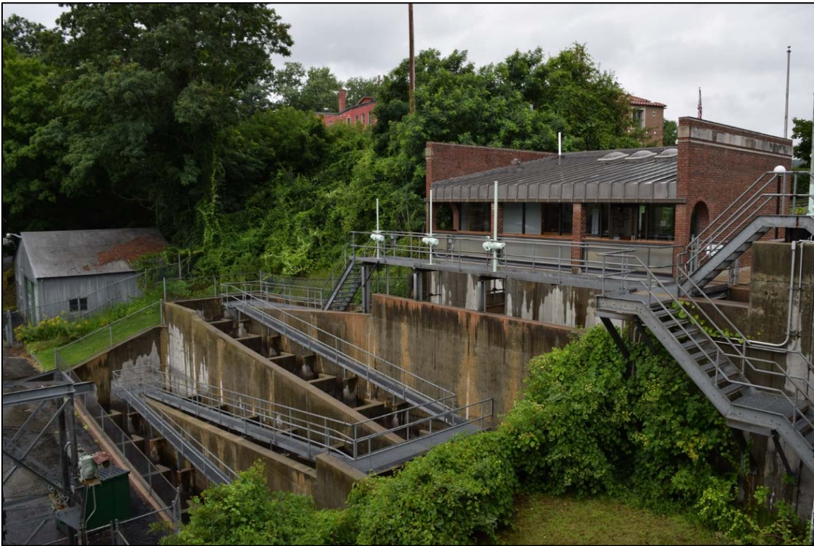
Photo 5-15. Bellows Falls Project, Visitors' Center and Fish Ladder, looking northwest.
