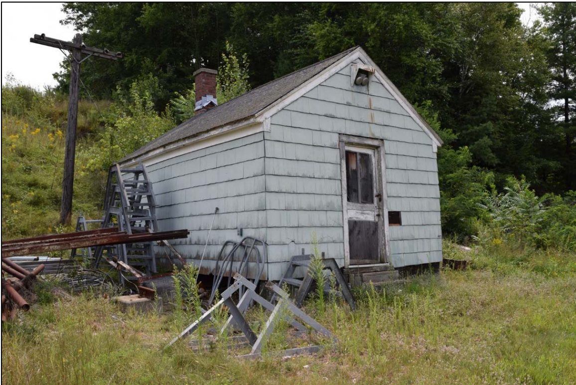
Photo 6-8. Vernon Project, Crew Shack looking southeast.
