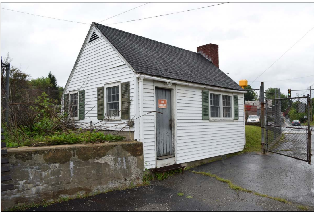
Photo 5-19. Bellows Falls Project, Crew Shack, looking northwest.
