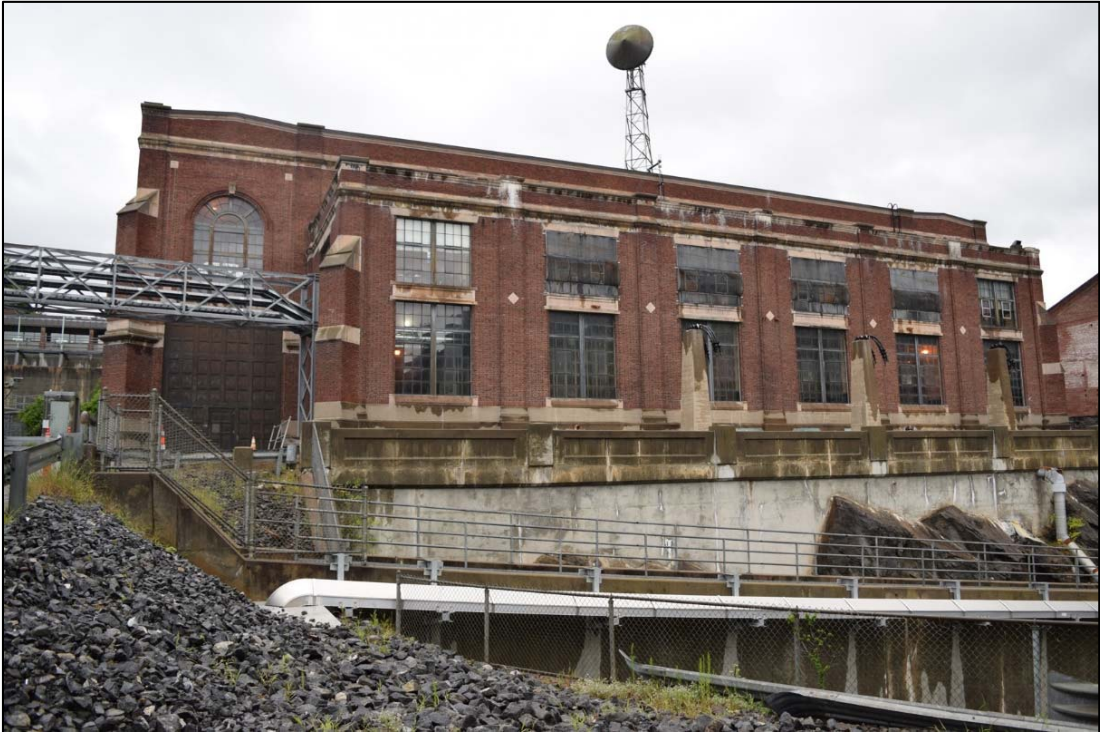
Photo 5-8. Bellows Falls Project, Powerhouse, looking north.
