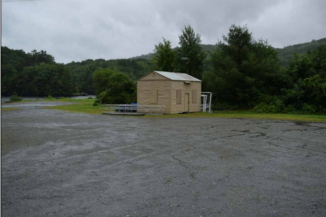
Photo. 4-18. Wilder Project, Oil Storage Shed, looking northeast.
