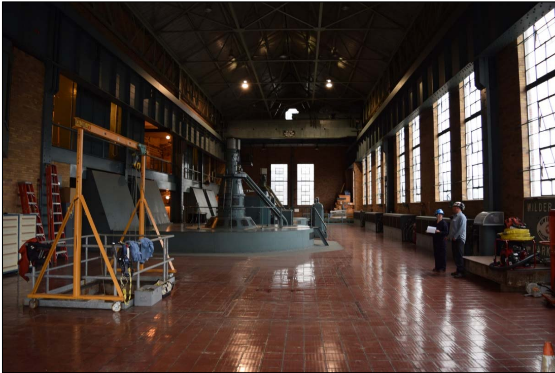
Photo 4-8. Wilder Project, Powerhouse, looking northeast.
