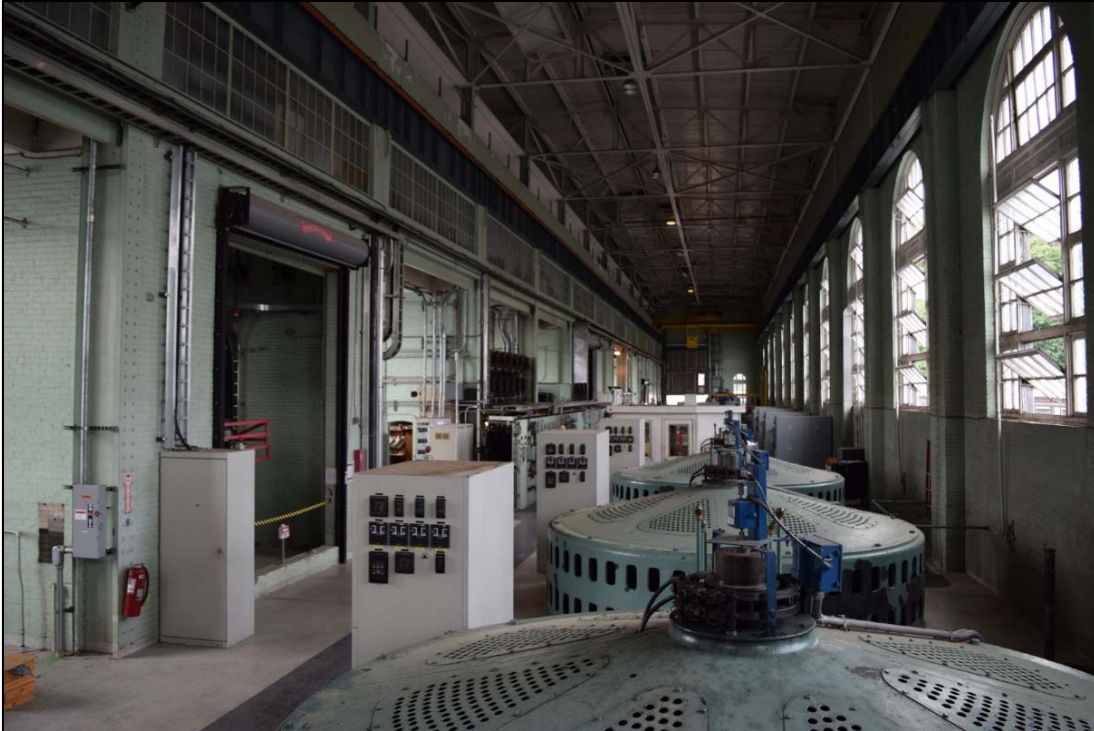
Photo 6-7. Vernon Project, Powerhouse generator hall, looking west.
