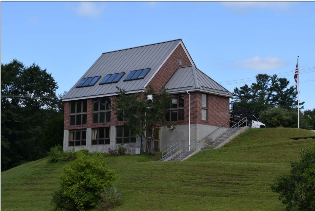
Photo 4-15. Wilder Project, Connecticut River Office, looking northwest.
