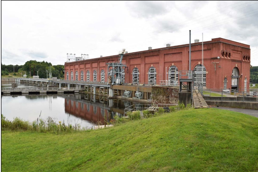
Photo 6-3. Vernon Project, Dam and Powerhouse looking southeast.
