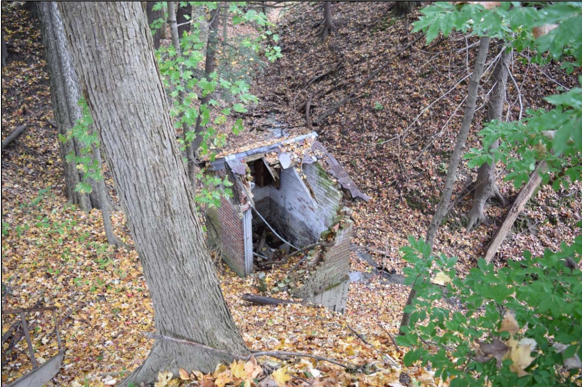
Photo 6-12. Vernon Project, Pump House, looking northwest.
