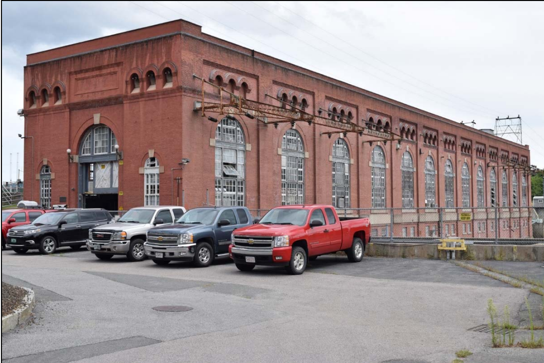
Photo 6-5. Vernon Project, Powerhouse looking northeast.
