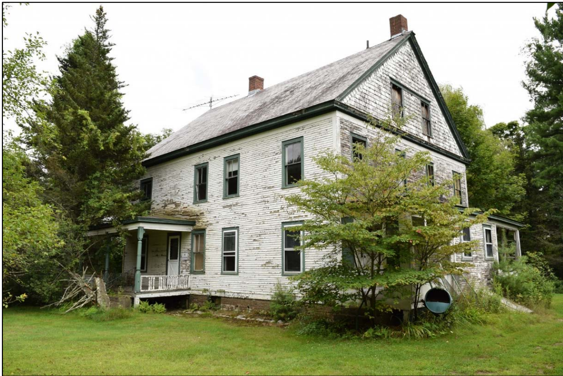
Photo 6-13. Vernon Project, Superintendent's House, looking southeast.
