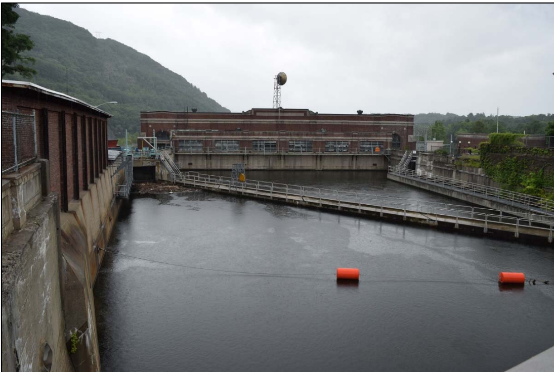
Photo 5-6. Bellows Falls Project, forebay of Canal and Powerhouse headworks building, looking south.
