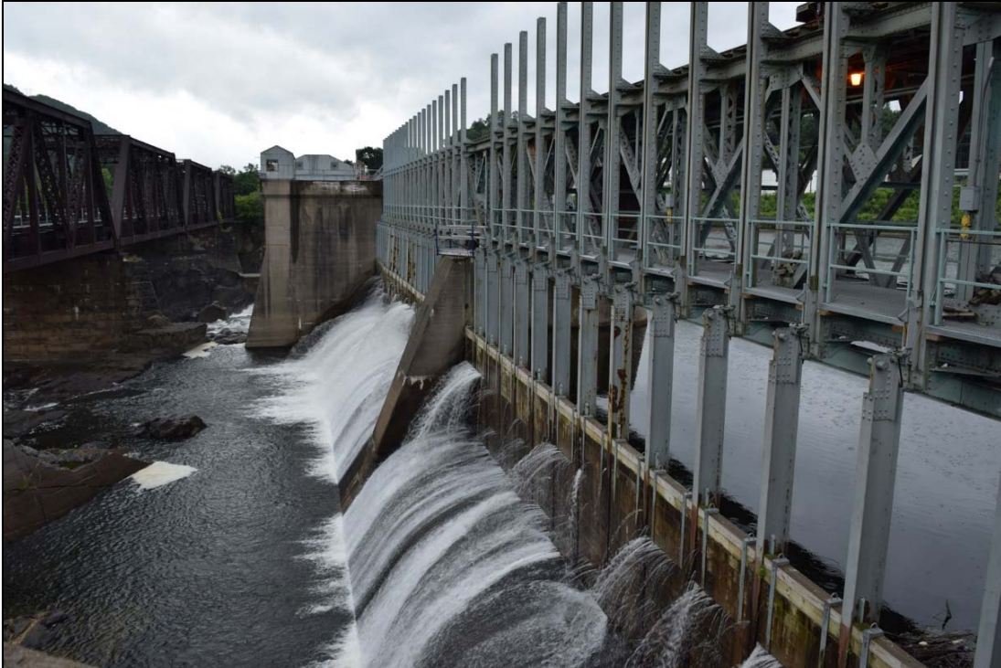
Photo 5-3. Bellows Fall Project, Dam spillway looking south from New Hampshire abutment.
