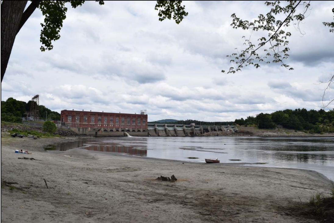
Photo 6-1. Vernon Project, general view looking north from Vermont riverbank.
