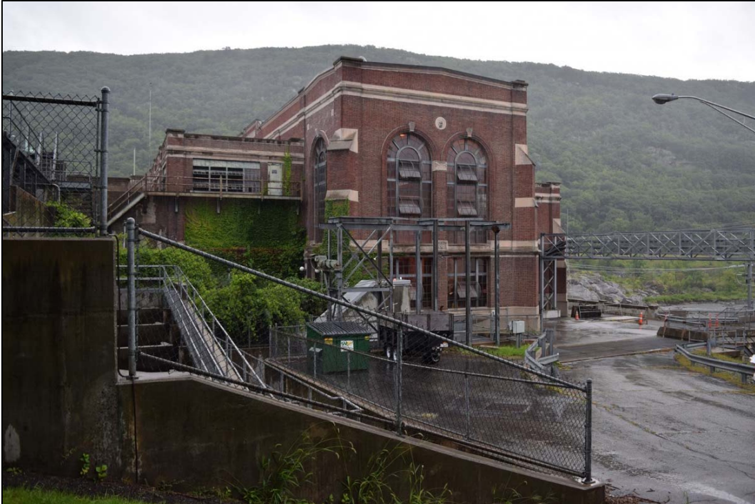
Photo 5-9. Bellows Falls Project, Powerhouse, looking east.
