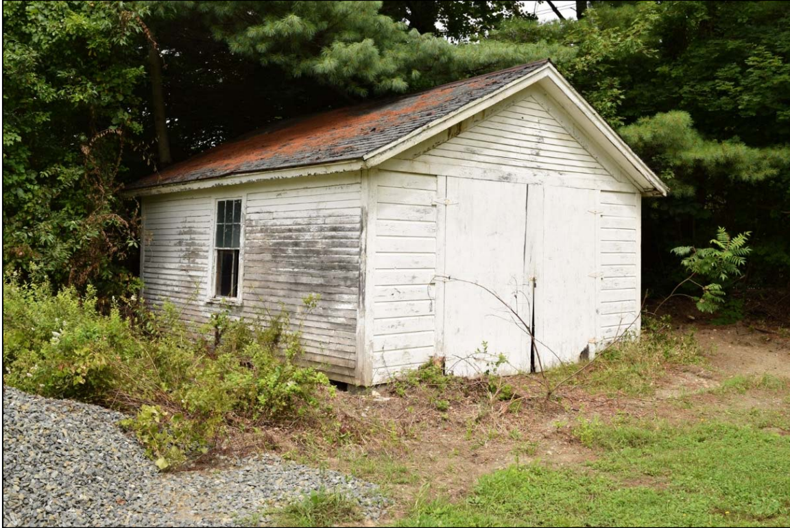
Photo 6-14. Vernon Project, Superintendent's Garage, looking northeast.
