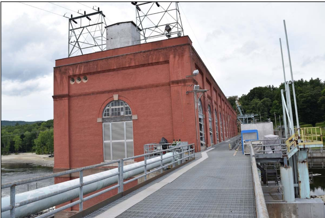
Photo 6-6. Vernon Project, Powerhouse looking southwest from dam.
