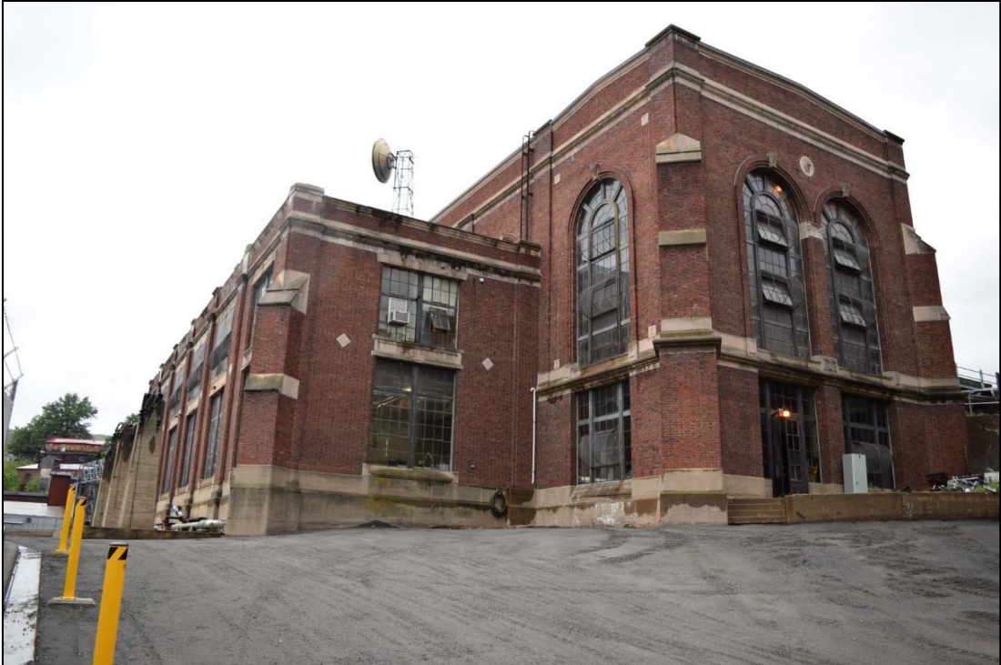
Photo 5-7. Bellows Falls Project, Powerhouse, looking northwest.
