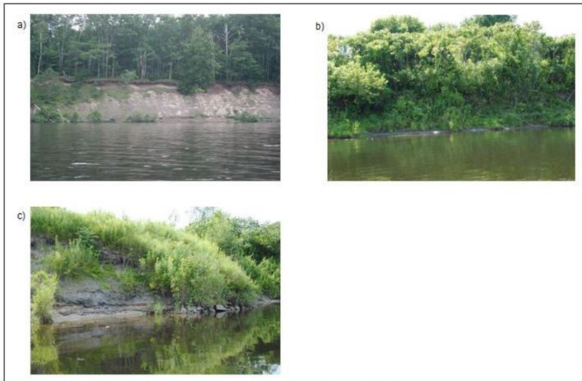
Photos of the unstable bank categories: a) eroding, b) vegetated eroding, c) failing armor.
