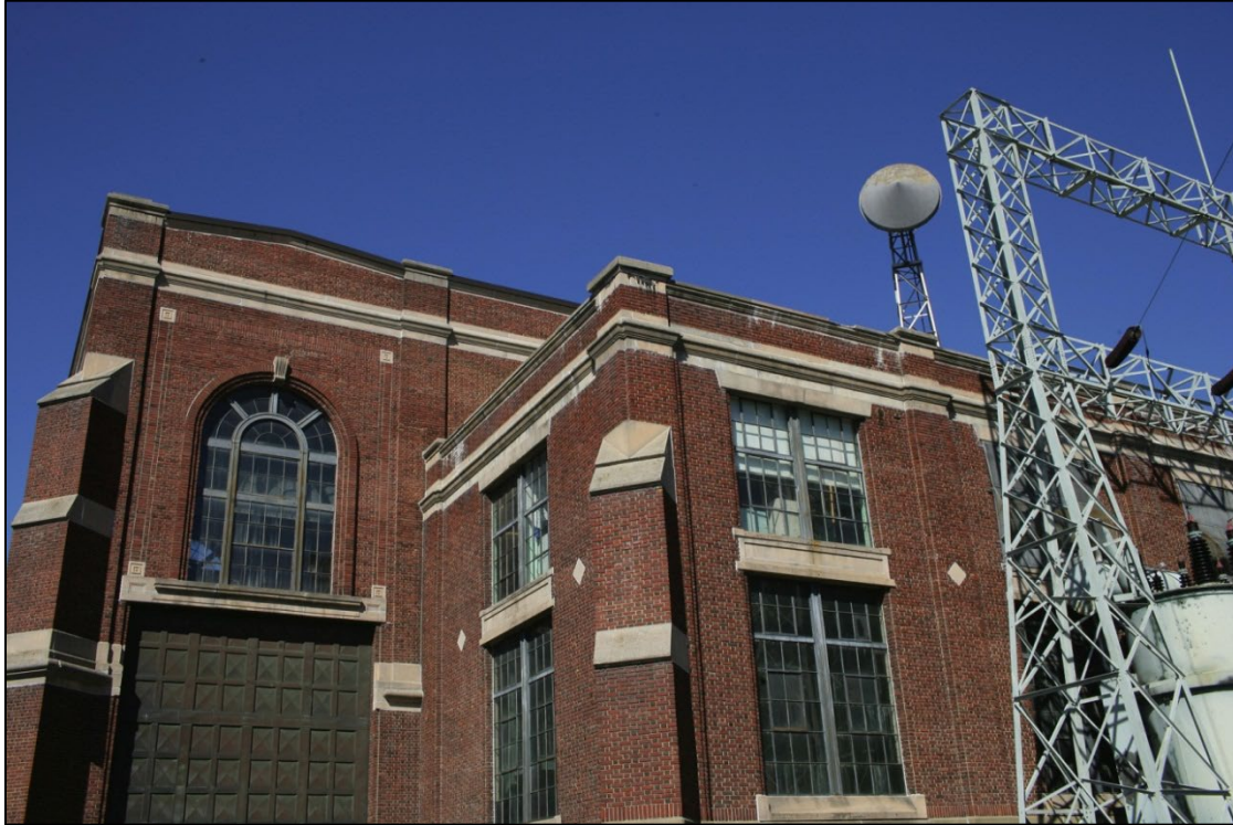
Figure A-5. Powerhouse.
