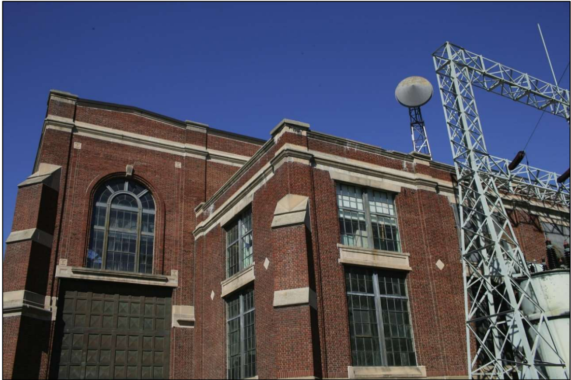
Figure A-5. Powerhouse.
