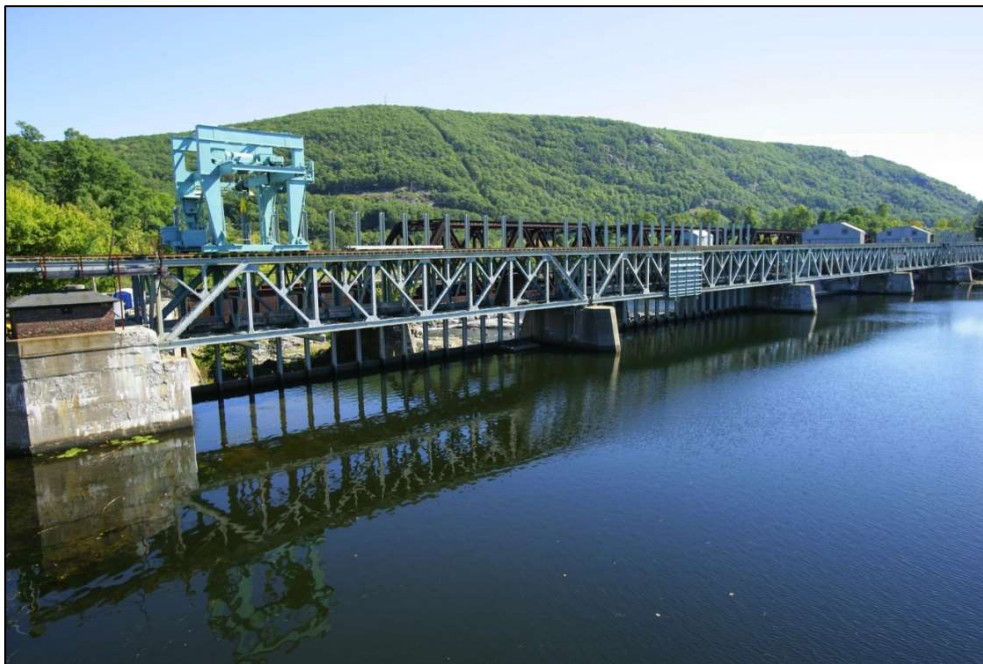
Figure A-3. Bellows Falls Dam (from upstream side).
