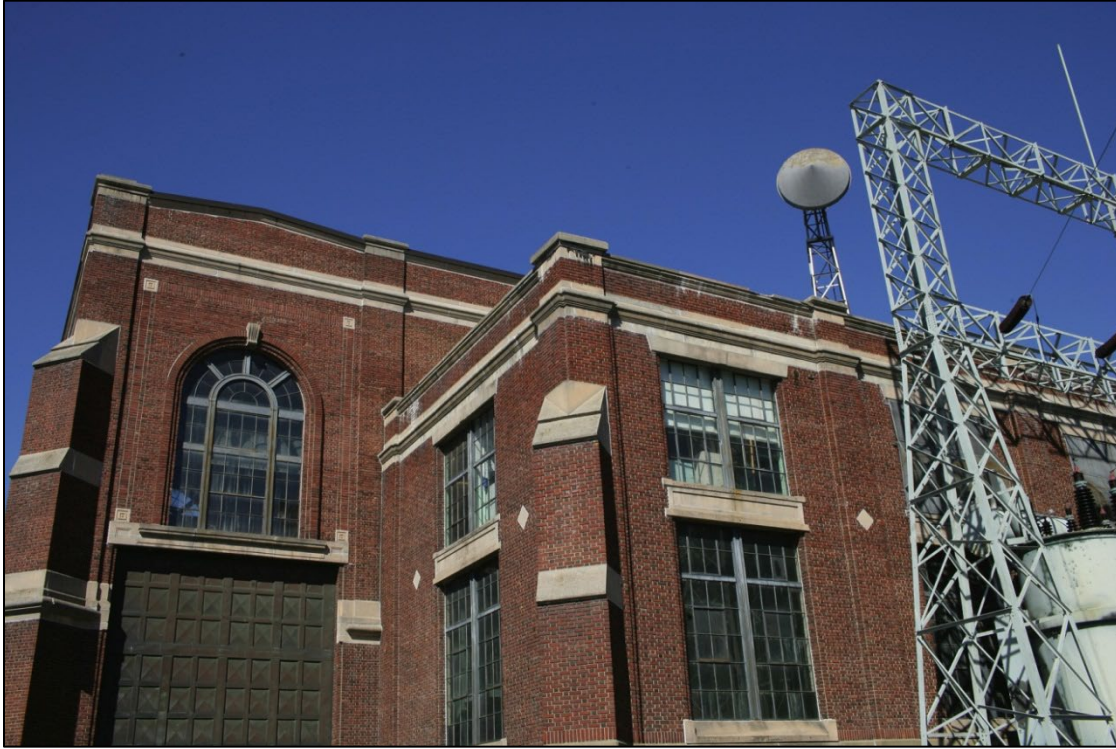
Figure A-5. Powerhouse.
