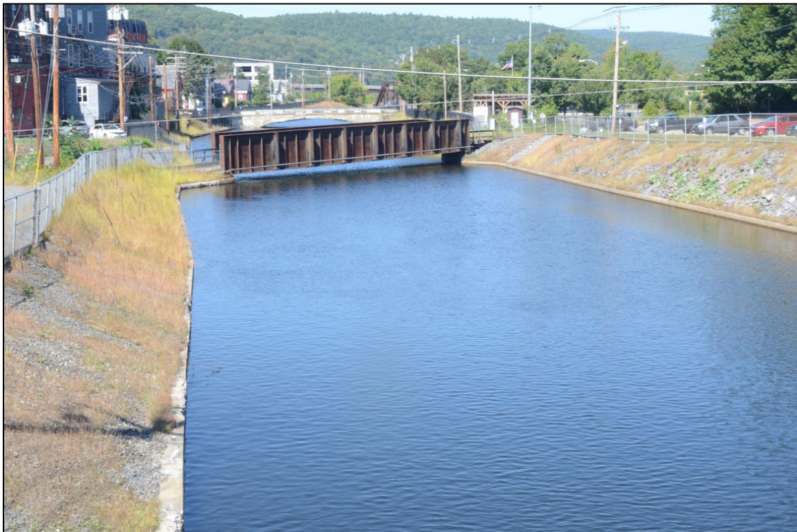
Figure A-4. Bellows Falls power canal (midstream, looking upstream).
