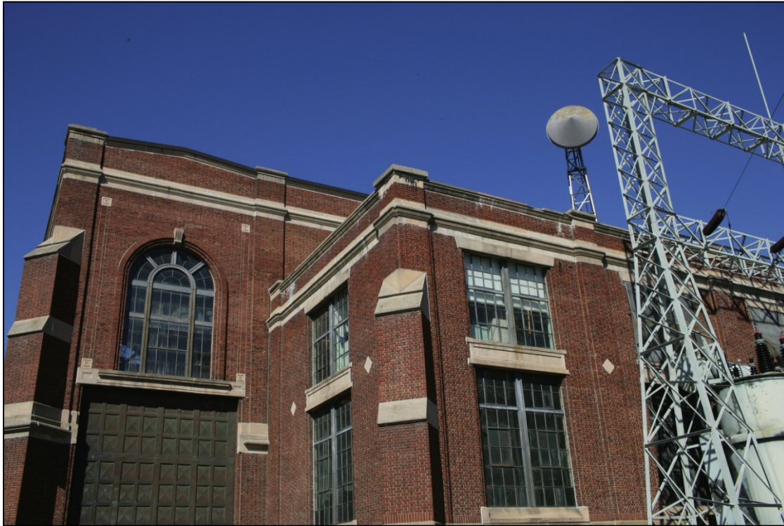
Figure A-5. Powerhouse.
