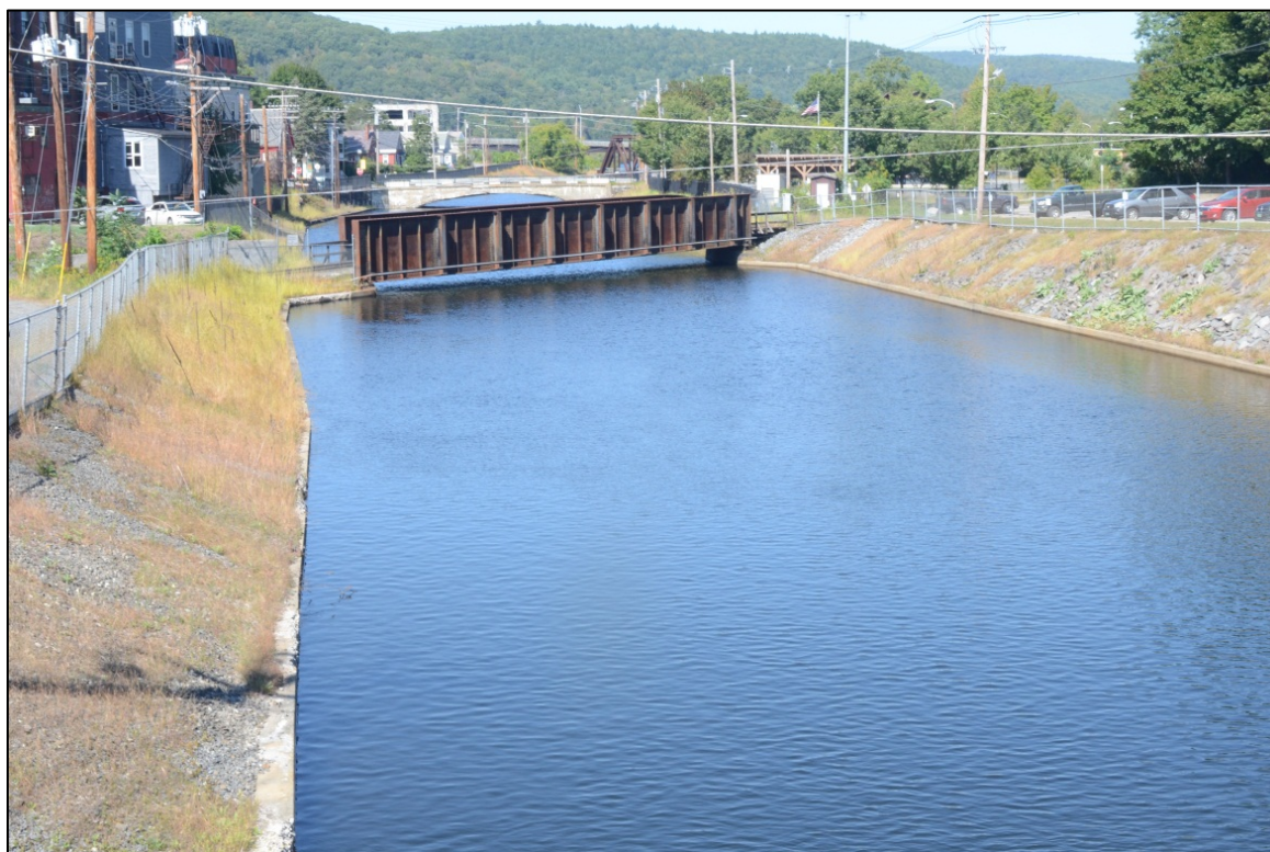
Figure A-4. Bellows Falls power canal (upstream end, looking upstream).
