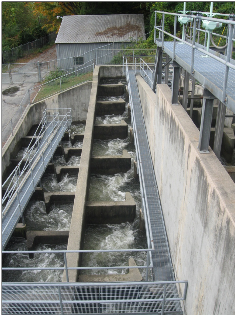
Figure A-9. Upstream fish passage facilities.
