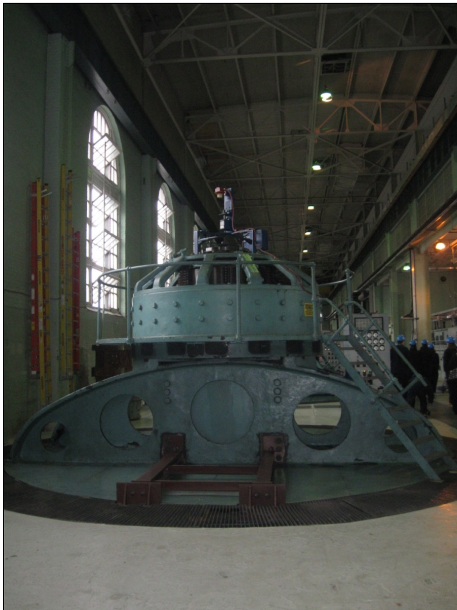
Figure A-4. Powerhouse, Unit No. 10.
