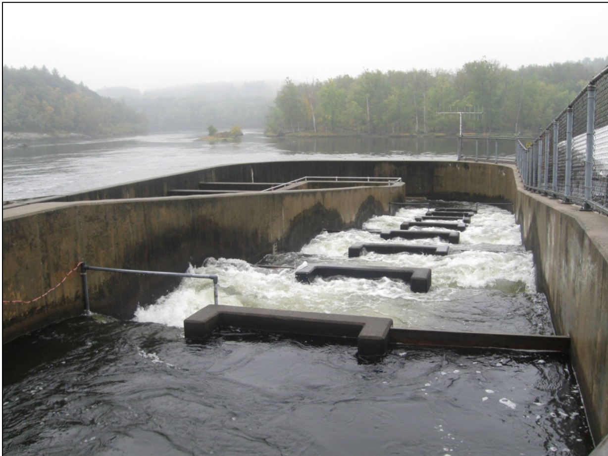
Figure A-6. Upstream fish passage facilities.
