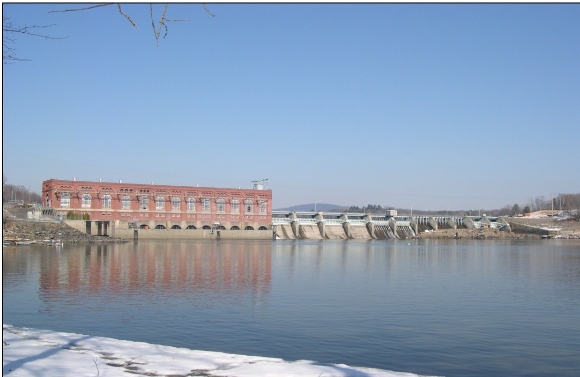
Figure A-3. Dam spillway and powerhouse (looking upstream).
