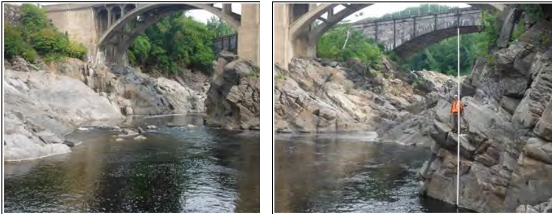
Photo 25. Bellows Falls Bypassed Reach; right and left channels under Vilas Bridge (top stadia rod 25 feet).
