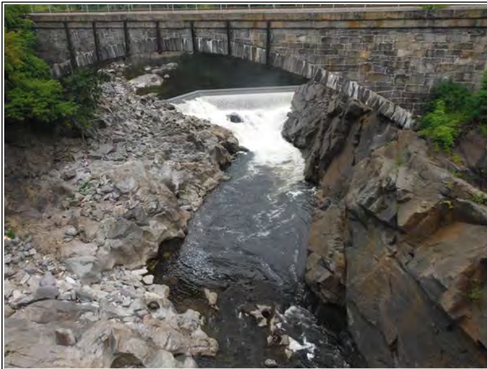
Photo 26. Bellows Falls Bypassed Reach; looking upstream right channel toward fish barrier from Vilas Bridge.
