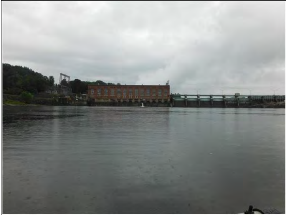
Photo 29. Vernon Reach; upstream view of dam and pool at ~3,500 cfs
