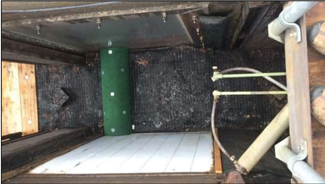
Figure 1.0-2. Counting window floor covered in plastic mesh and speed bump installed.
