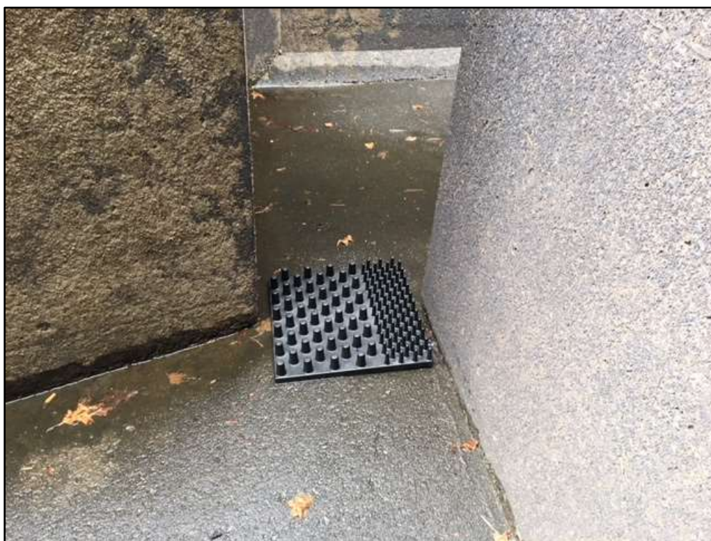
Figure 1.0-5. Eel tile placement in serpentine section upstream of the counting window.
