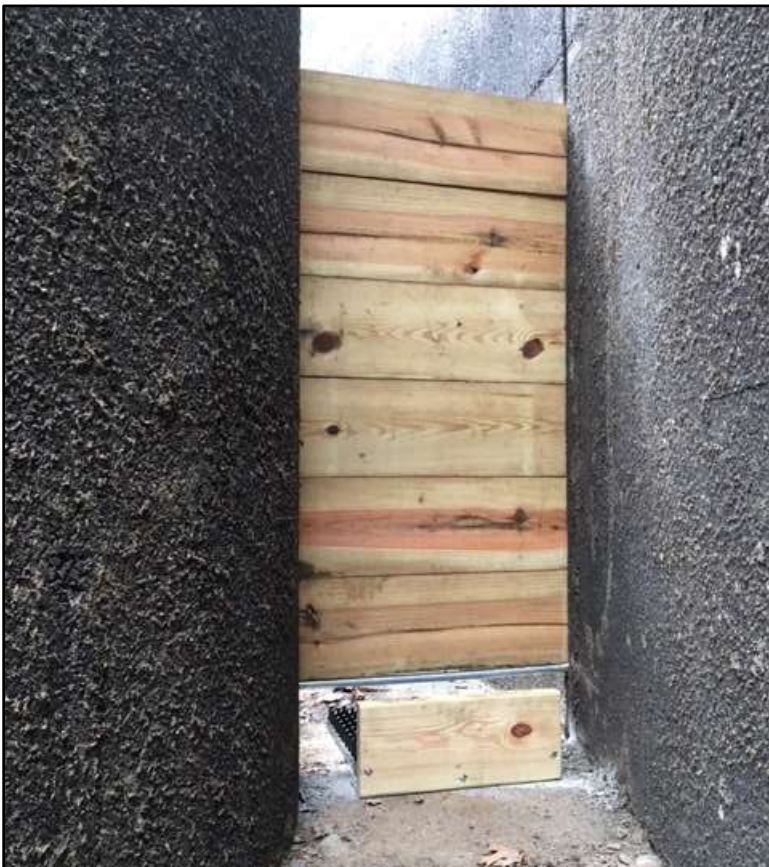
Figure 1.0-3. Exit Weir looking downstream with eel tile and upstream baffle.
