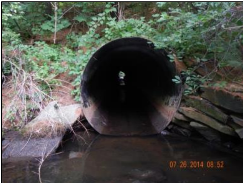
Culvert near upstream extent of project-affected area associated with Site CT-B-3.35 as determined by visual observations, 2014.
