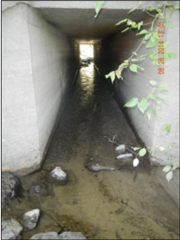
View looking upstream through tunnel at site CT-W-1.06.
