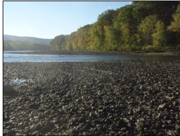
Photo C.87. View across Study Site 08-T14, facing south across the delta bar. The Saxtons River is visible in the midground of the photograph, and its confluence with the Connecticut River is visible at the left side of the photograph. (Stantec 10/9/14)
