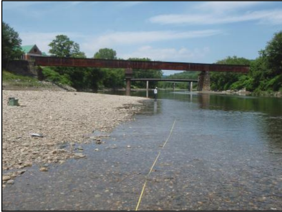
Photo C.75. View across Study Site 08-T02, facing upstream from the start (downstream limit) of Transect 3. The alignment of Transect 3 is indicated by the tape measure visible in foreground of photograph. (Stantec 07/12/14)
