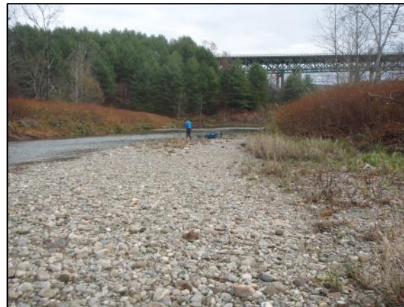
Photo C.82. View downstream across Study Site 08-T12 along Williams River with Interstate 91 Bridge in background. (Stantec 10/31/14)
