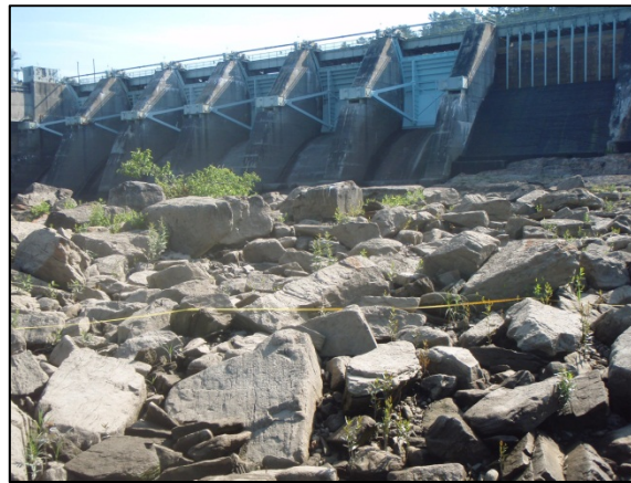
Photo B-1. View across Study Site 08-M01, facing upstream towards Wilder Dam. The location of Transect 1 is indicated by the tape measure visible in the midground of the photograph. (Stantec 07/12/14)
