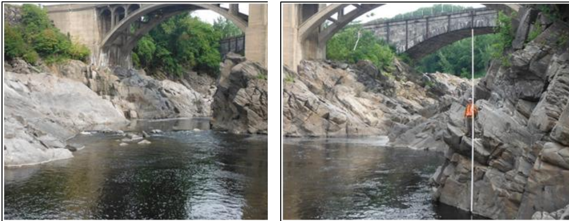
Photo 25. Bellows Falls Bypassed Reach; right and left channels under Vilas Bridge (top stadia rod 25 feet).
