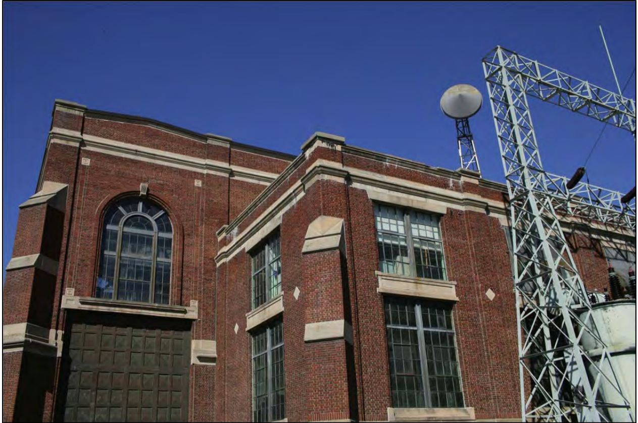
Figure 2.3-5. Bellows Falls powerhouse.
