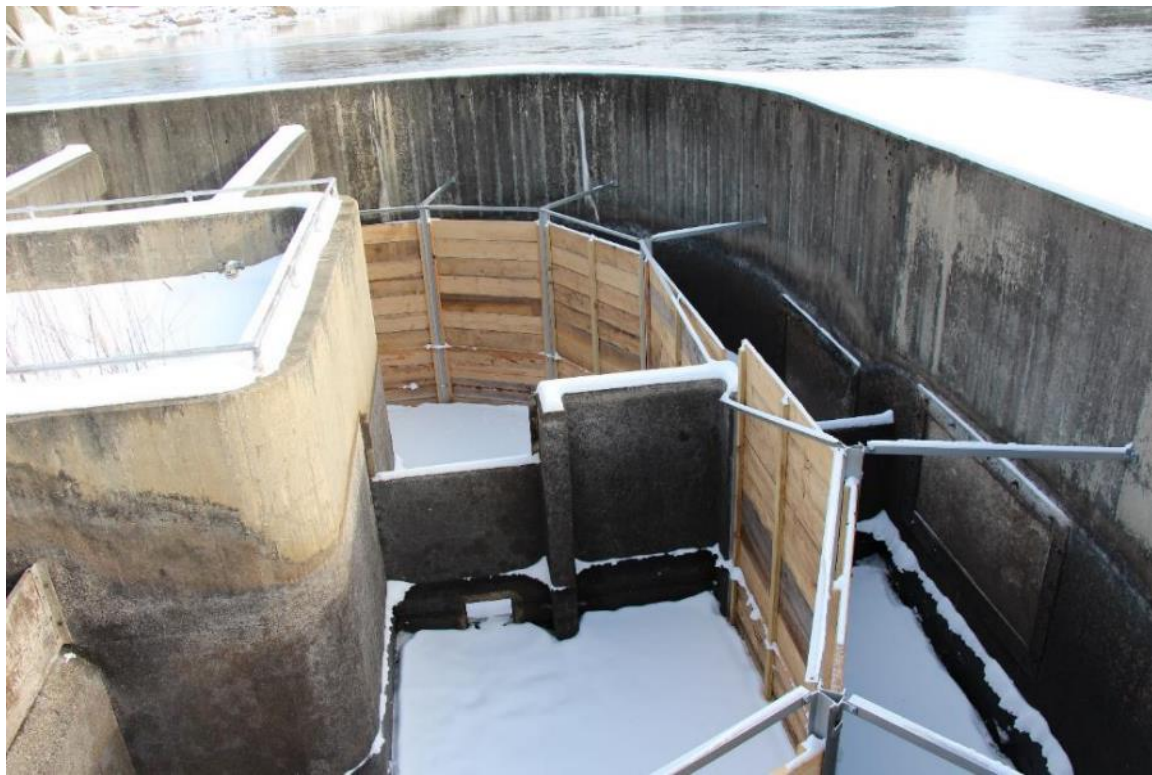
Figure 3.6-21 Partition wall installed at the Vernon fish ladder prior to the 2019 fish passage season.
