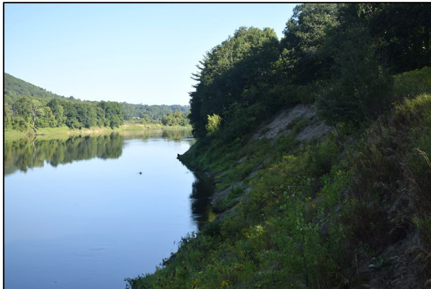
Figure 1. The 40-foot high bank at the Lipfert site is composed of glacial outwash sediments.
