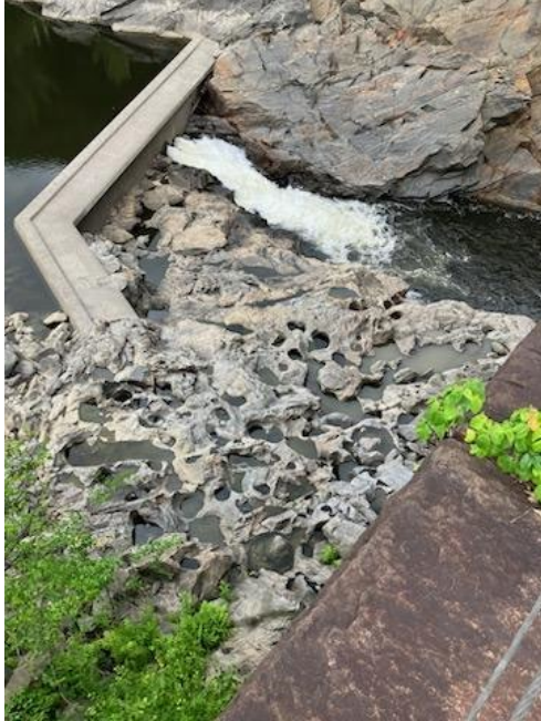
Photo of water passing “under” the salmon dam during low flow conditions. Photo take July 7, 2022 by Annette Spaulding.
