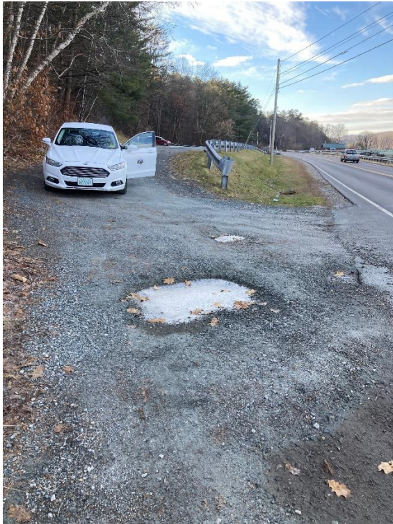
* Poor drainage and long established potholes. Photos taken December 2023.
