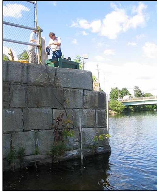
Photo 1. Hydroacoustic transducer mounts, power supply, sounder, and computer network component installation at the Anson Project, Madison, ME.
